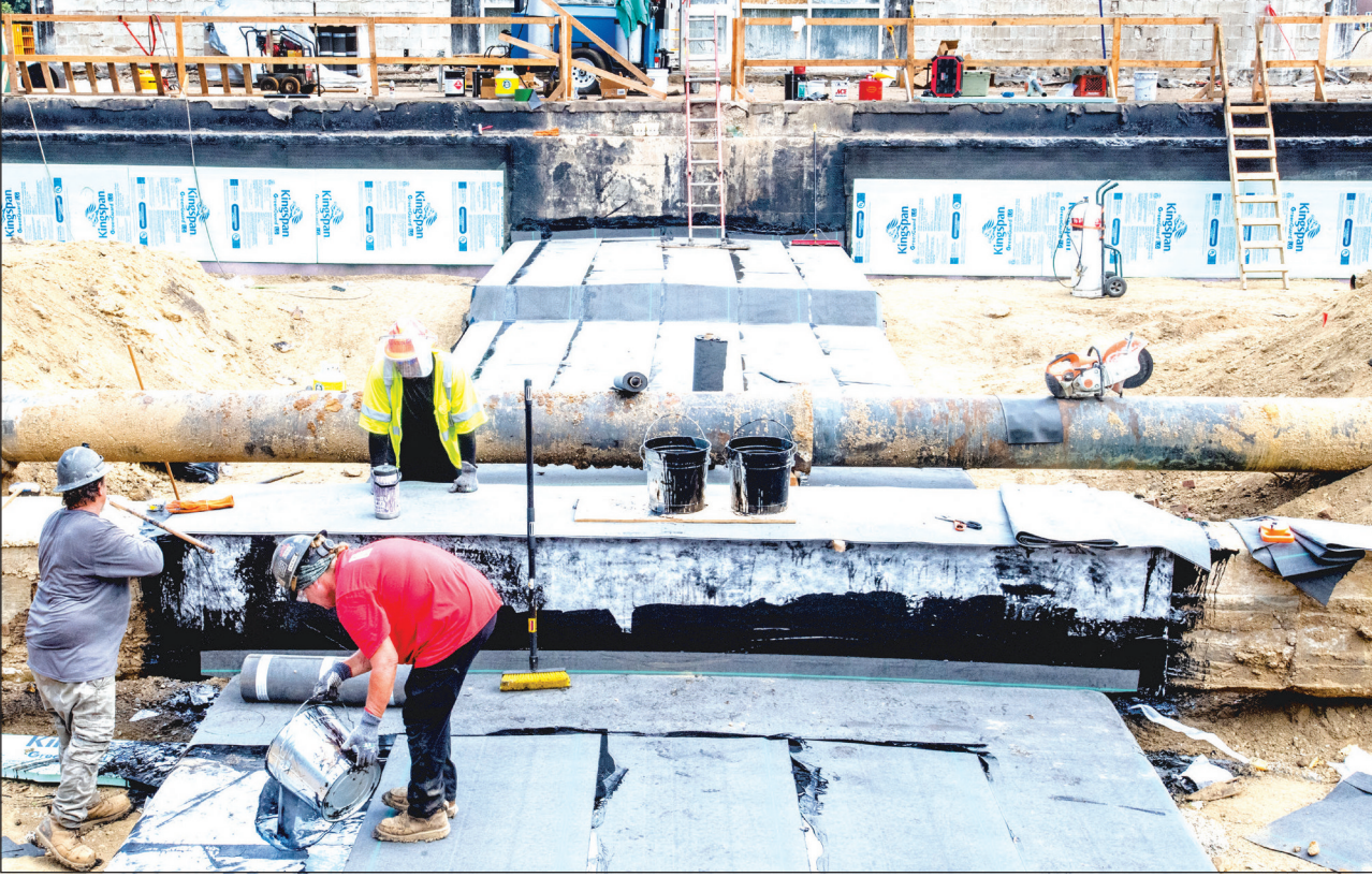
AUG. 14: From left, Tim Hafele, Jennifer Hafele (in red) and Jay LaRue, all employees of Williams Bros. of Peoria, pour tar and lay tar paper on top to cover the roof of the tunnel leading from the University of Illinois Main Library to the Undergraduate Library on campus in Urbana. The work was part of renovations to turn the underground area into the Archives and Special Collections building.
