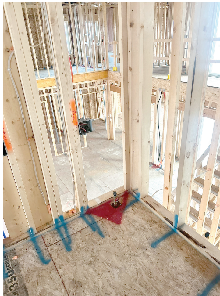
Dionne Clifton's new home in southeast Urbana is all studs, pipes and wiring during the framing process, as shown from the second floor looking down to the first. Clifton had a hands-on approach in the process from site selection to design and through construction.
