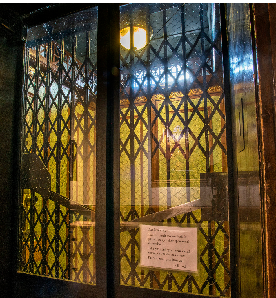
ABOVE: The Buzard Pipe Organ Builders building at 112 W. Hill St. in downtown Champaign is shown in the early 1980s, when it still had a roof over the front patio. BELOW: The 1902 Otis Dual Speed elevator still has the original car, scissor gate and hoistway.
