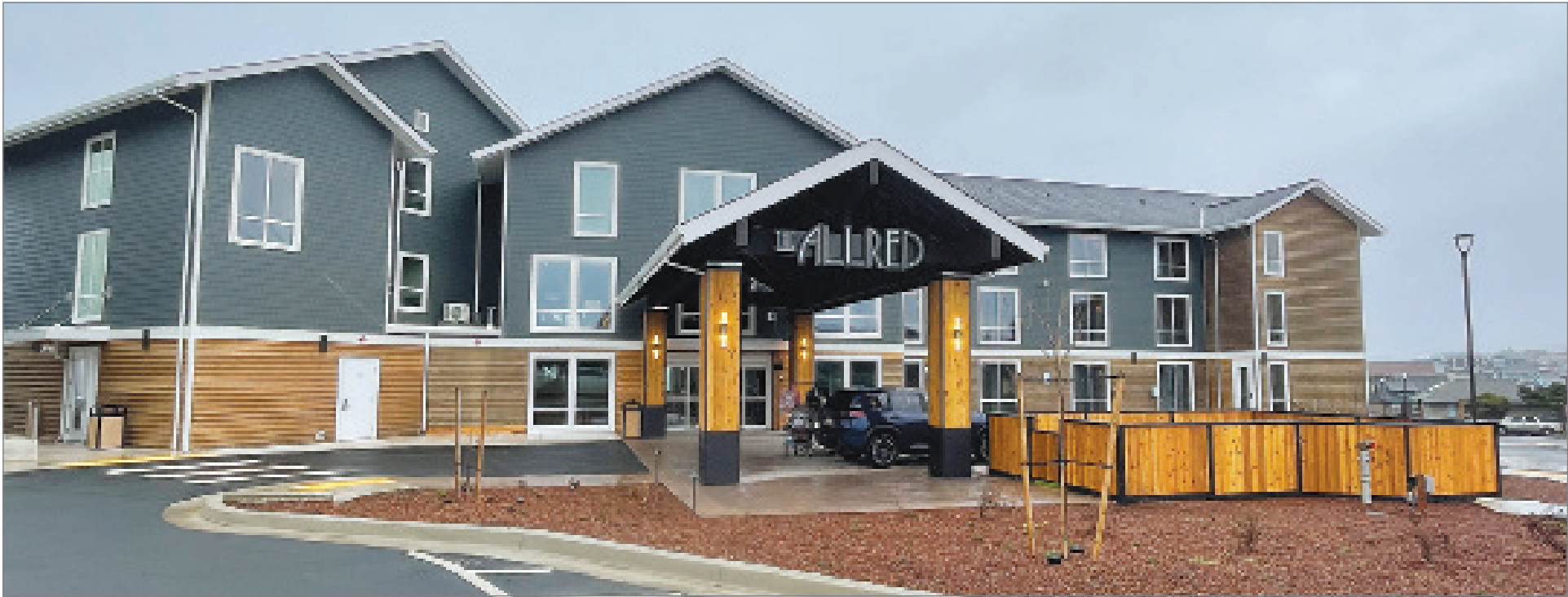
The renovation, expansion, and rebranding of the Whaler Motel to the Allred Hotel has been completed. The hotel is located at 155 SW Elizabeth St. in Newport. (Photo by Steve Card)
