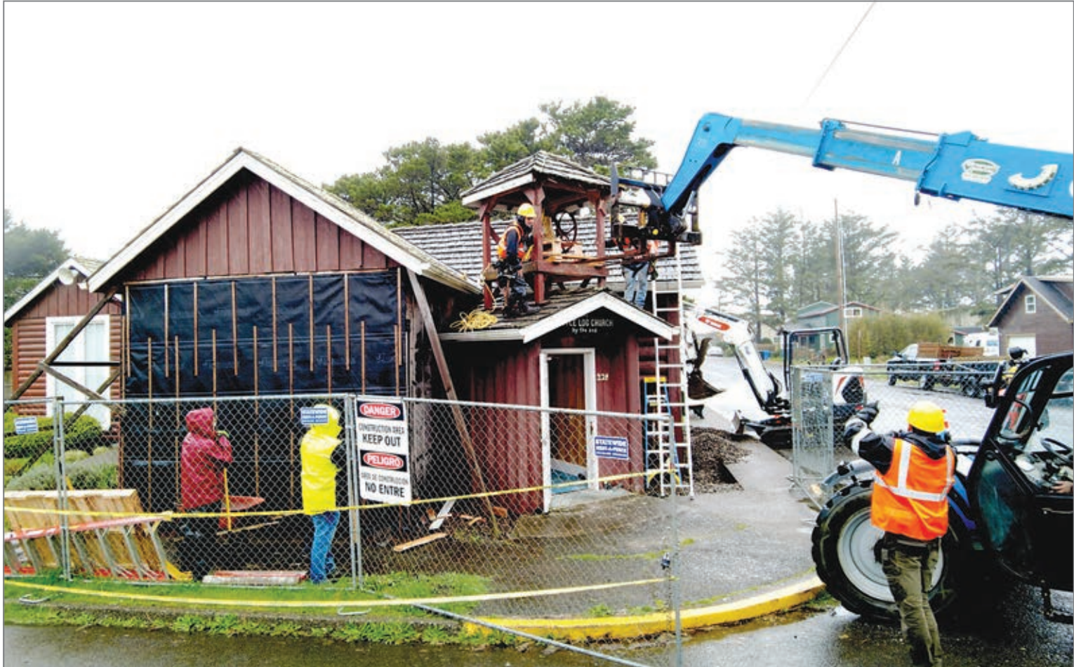
The bell was removed from the Little Log Church & Museum in Yachats on Thursday, March 20, as part of a renovation project being done by Top to Bottom Contractors of Newport. (Photo courtesy of Dave Wilson/West Coast Drone Services)
