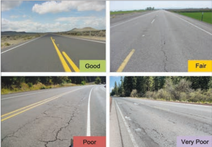
ODOT uses this photo illustrating the highway deterioration. (Courtesy photo from ODOT)
