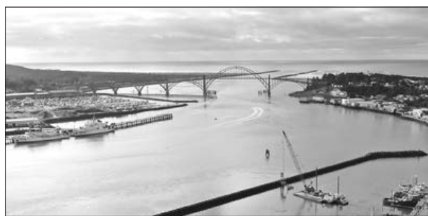
The Yaquina Bay Bridge restoration is project is complete, according to the Oregon Department of Transportation. Restoration was crucial to keep the bridge safe and in good working order, ODOT officials said. (Photo courtesy of the Oregon Department of Transportation)
