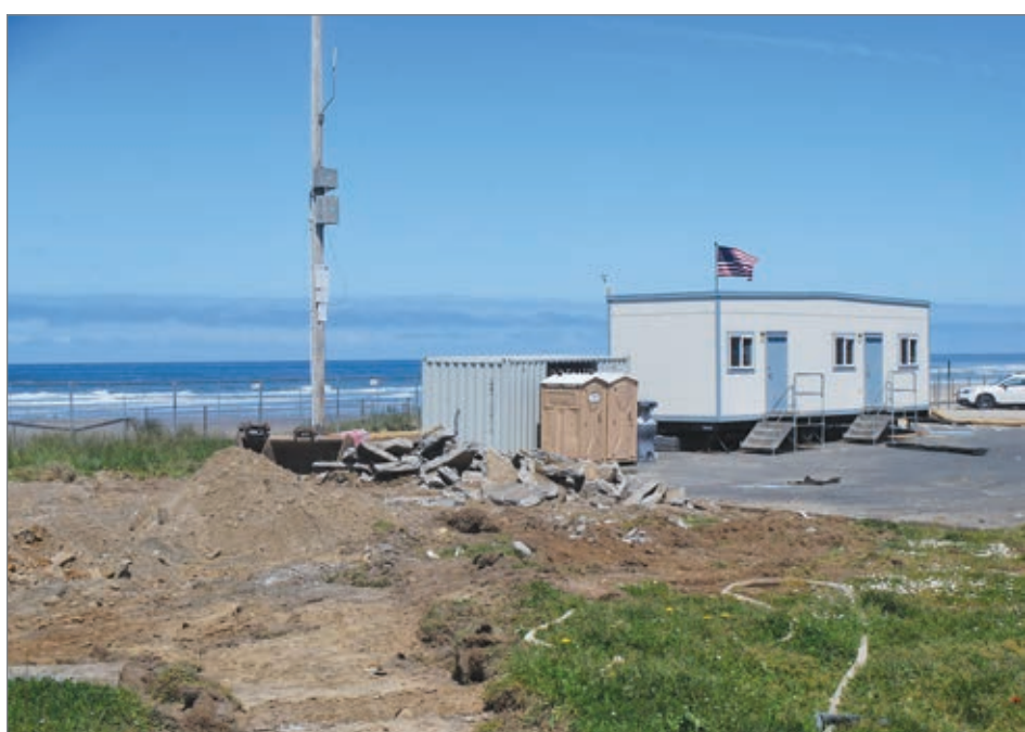
All that was left May 11 at the D River Wayside restroom building was rubble after construction crews removed the structure. (Photos by Jeremy C. Ruark / Lincoln County Leader)
