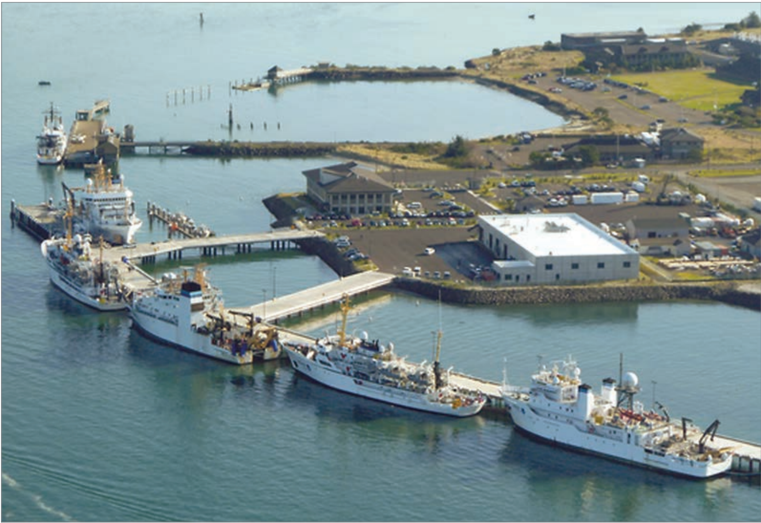
NOAA Marine Operations Center in Newport. (Courtesy photo from Wikimapia)
