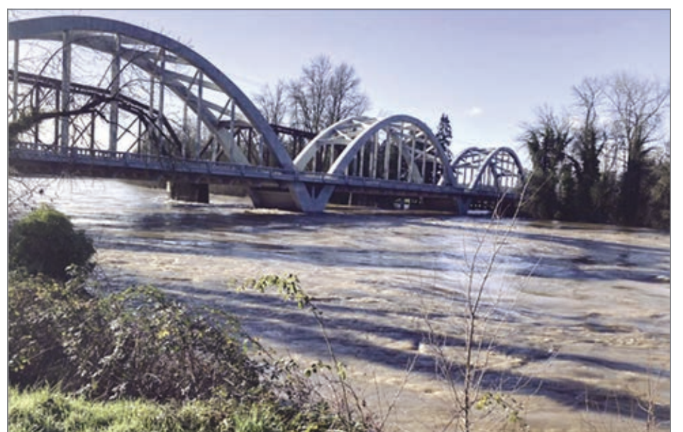
The December storms caused widespread damage across nine Oregon counties, including Lincoln and Tillamook counties. (Courtesy photo)
