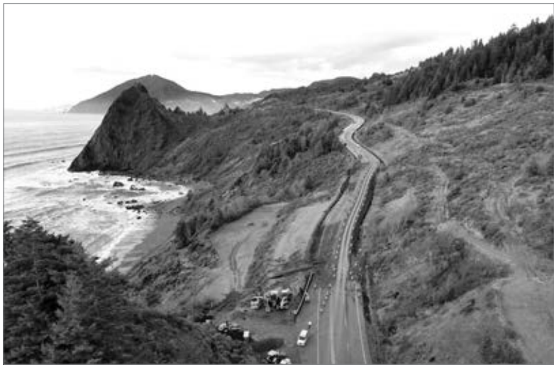
An aerial view of the Arizona Slide, a landslide along U.S. Highway 101 near Port Orford and Gold Beach. Oregon Department of Transportation. (Courtesy photos from the Oregon Transportation Department)
