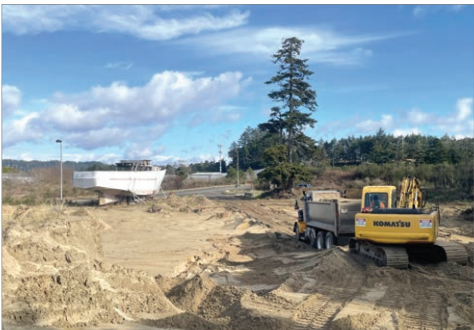
Sand is loaded onto trucks at Southeast 40th Street and Highway 101 for use as fill material for a building project in north Newport. (Photo by Steve Card)
