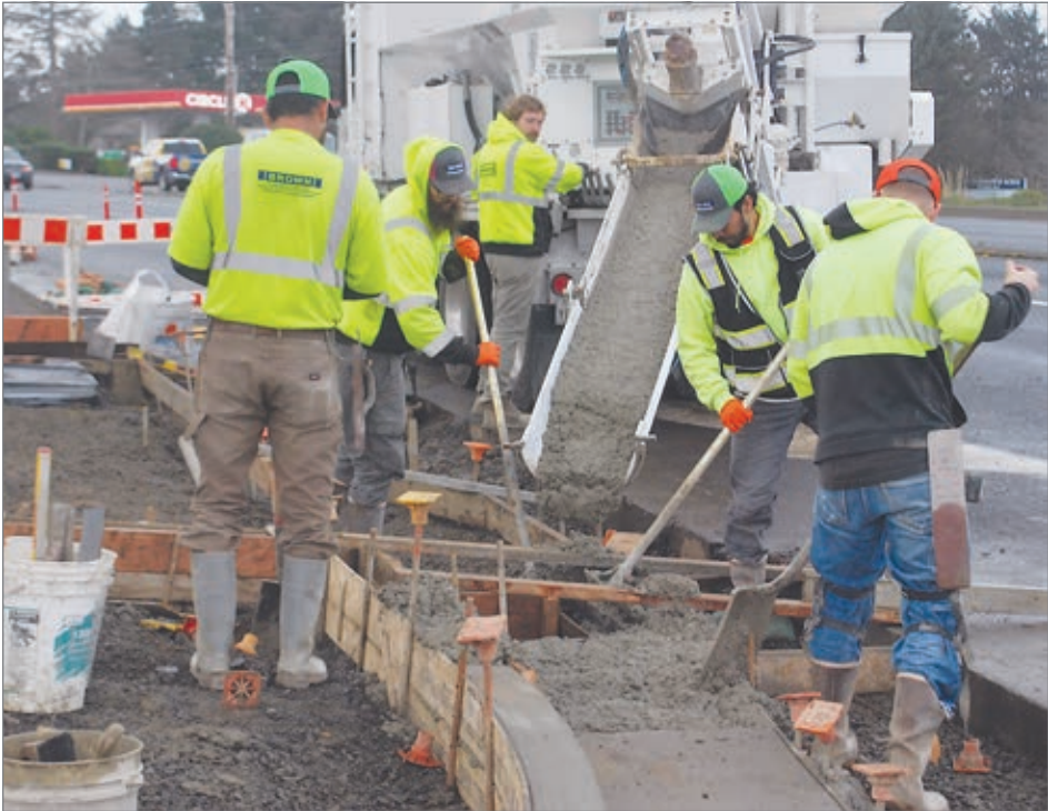
ODOT crews work to repair and replace the curb ramps along Highway 101 at Logan Road in Lincoln City. Jeremy C. Ruark / Lincoln County Leader.
