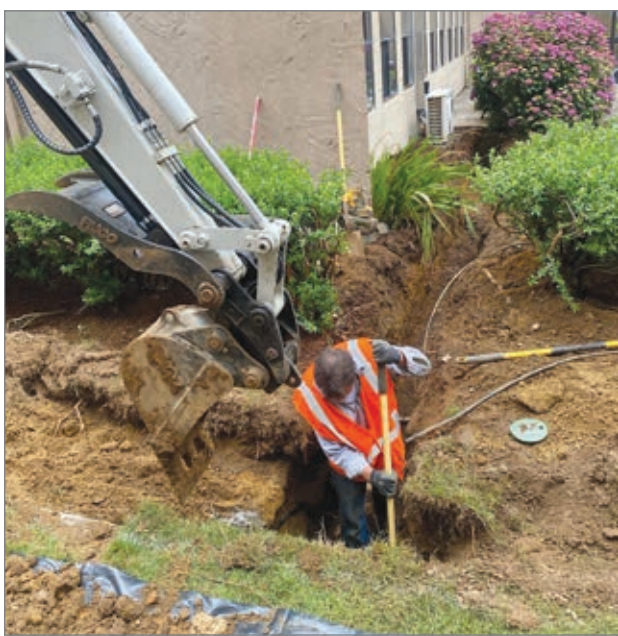
Local service providers Rau Plumbing and JSC Contractors rearranged their schedules over the major holiday weekend to complete the emergency repair. By Monday morning, the excavation area had been filled and covered, required inspections had been approved by the City of Newport. (Courtesy photos)
