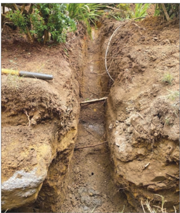
The repairs were made in the Heather Hosey Memorial Garden, located immediately outside the Lincoln County District Attorney's Office windows. involved for responding quickly, protecting public access, and completing the repair for under $10,000."
