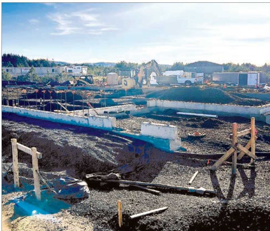
Footings are in place for the new Lincoln County Animal Shelter in Waldport. The pouring of cement for the foundation was scheduled to being on Monday of this week. (Courtesy photo)
