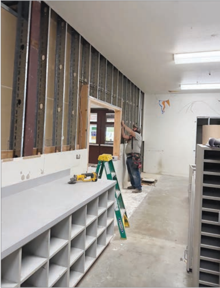
A worker on the job at the Career and Tech Education wing remodel project at Taft 7-12 Middle High School. (Courtesy photos)
