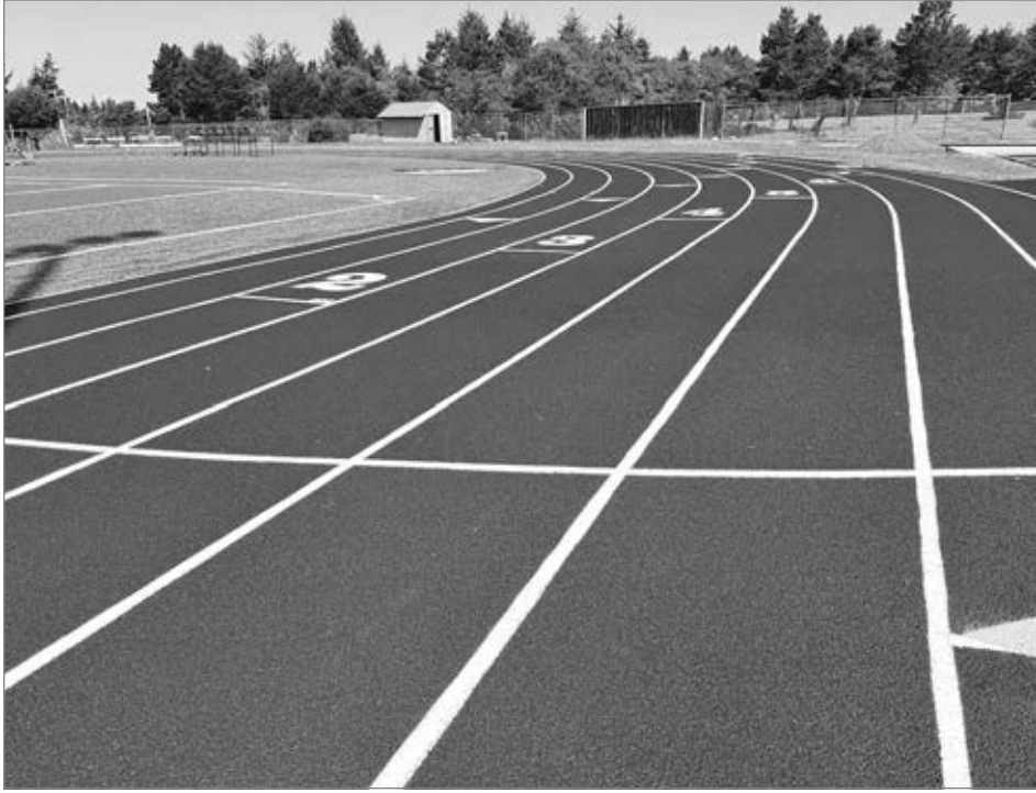
A new athletic track at Taft 7-12 Middle High School has been completed.
