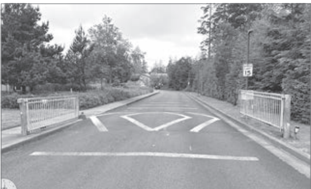
This permanent asphalt speed hump is the type that will replace all of the pre-fabricated speed humps currently installed on Oceanview Drive. (Courtesy photo) version is $75,000. Beatty told the city council the project still needs to go out for bid to identify a contractor. He also said because the existing speed humps are removable, they can be repurposed.
