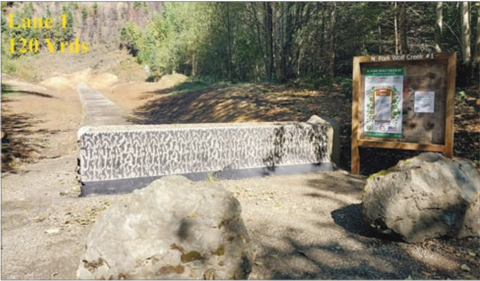
Thanks to the non-profit Trash No Lands who put more than $30,000 toward improvements at Wolf Creek Shooting Lanes recreational shooters now have longer lanes, gravel staging areas, gravel walkways, new informational signs, repainted Jersey barriers and improved backstops. (Courtesy photos)
