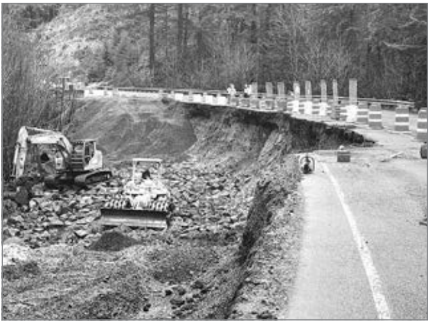
Highway 6 near milepost 35 was fully closed Jan. 4 in both eastbound and westbound directions near milepost 35 due to construction to repair the washed-out section of roadway. One temporary lane was open late that evening. (Courtesy from the TCSO)
