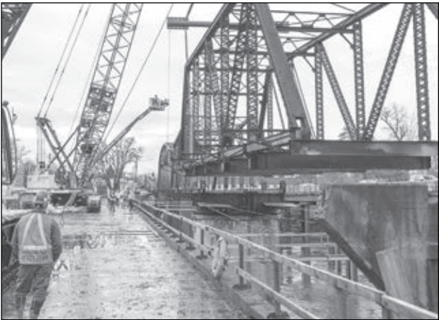
Construction crews use a crane to remove the old Van Buren Bridge in Corvallis in preparation for the new bridge. (Photo courtesy of ODOT)
