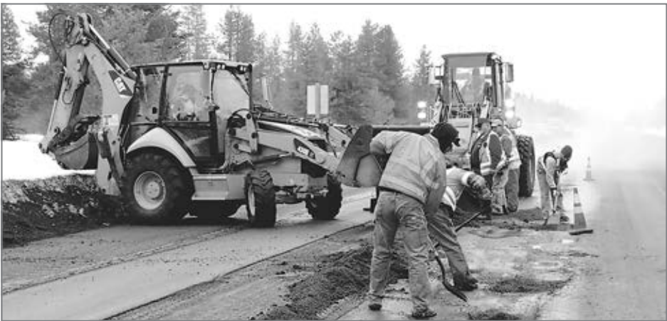
Oregon Department of Transportation workers fill a pothole on U.S. Highway 97 near Chemult in 2016. Courtesy from the Oregon Department of Transportation/Flickr)
