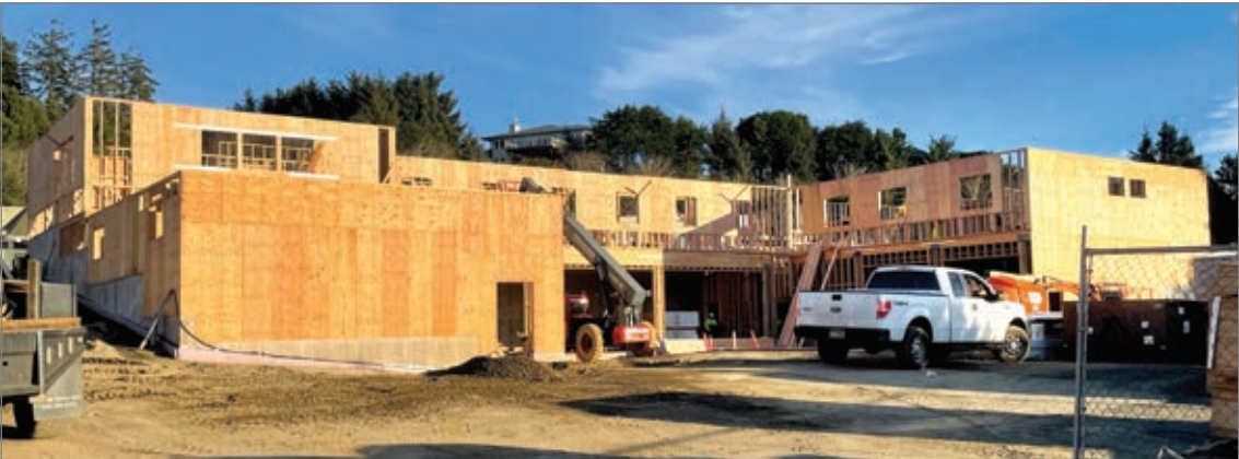
A new building is being constructed at the end of Northeast 73rd Street in Newport, just east of the Oregon State Police office, that will become the new home of the Oregon Department of Forestry Newport Unit. It will also be the site of the Newport Fire Department's north station. (Photo by Steve Card)
