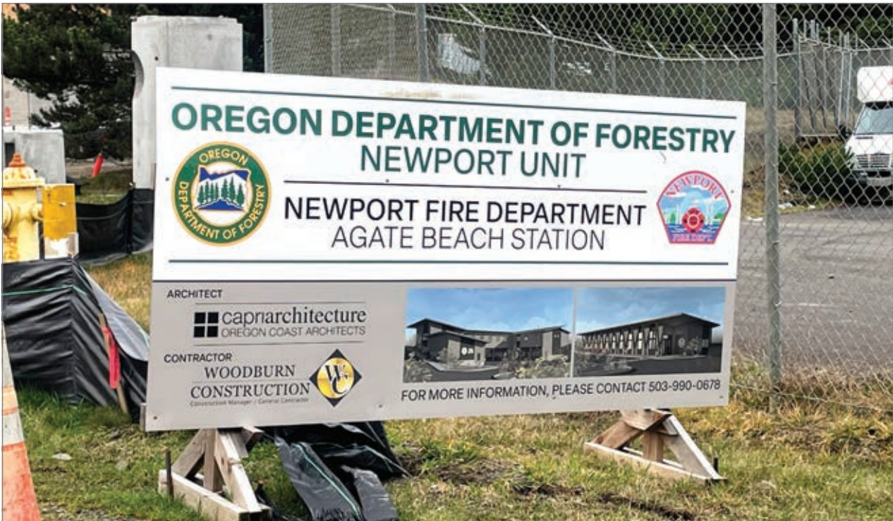
This sign marks the location of the Oregon Department of Forestry’s new building in north Newport, which is expected to be completed this fall. (Photo by Steve Card)
