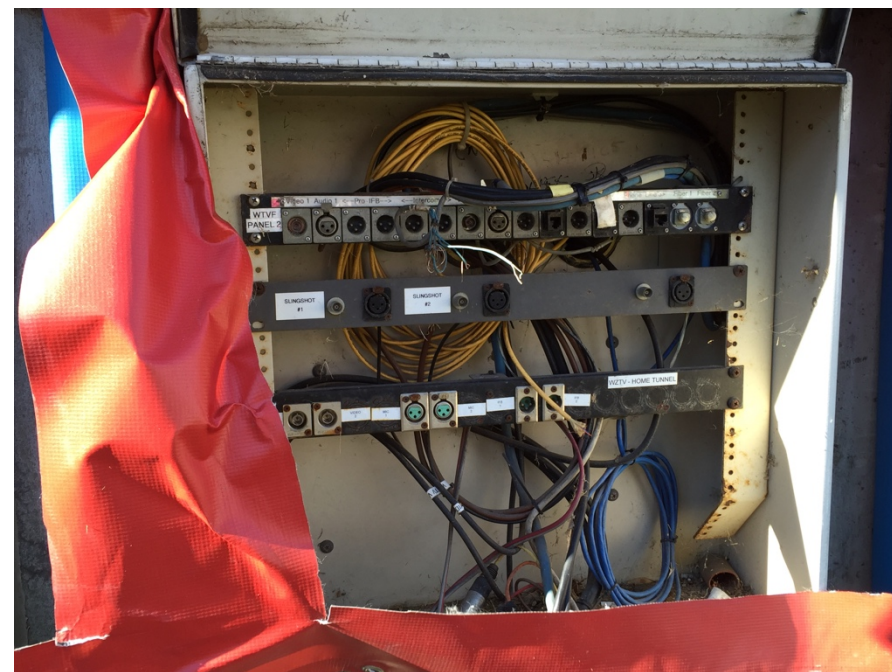
Rusted and corroded coax and audio connections in corroded connection box
