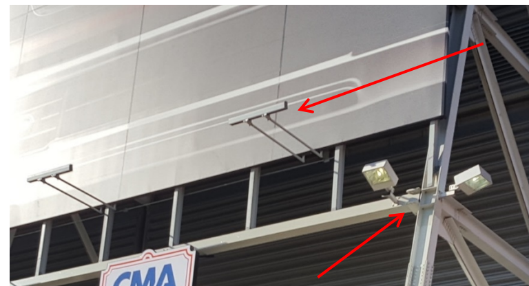
Metal Halide and LED Luminaires (on during the day)
