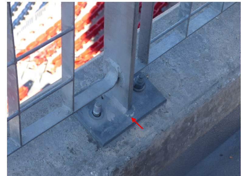
Missing nut on handrail base plate on club level
