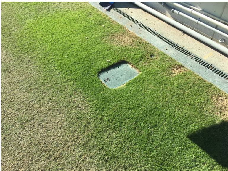
Perimeter Irrigation Remote Control Valve
