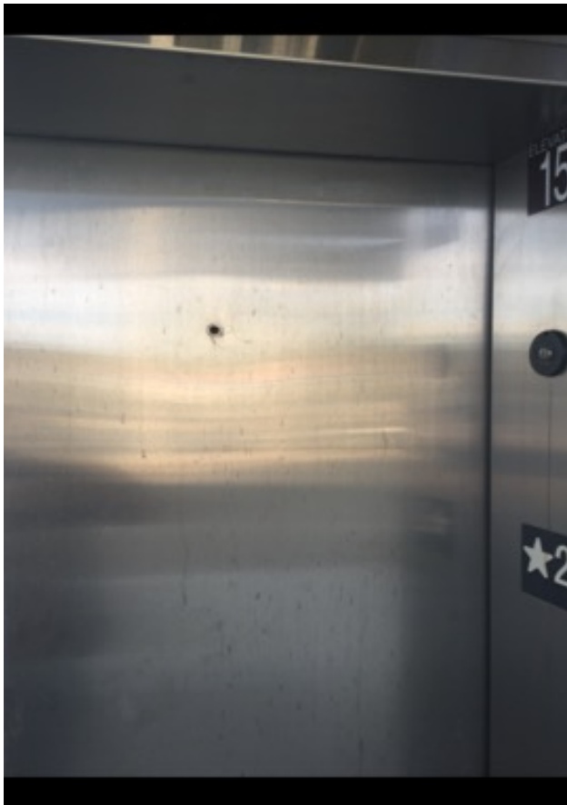
Weather Damaged Hall Door Entrances on Express Units
