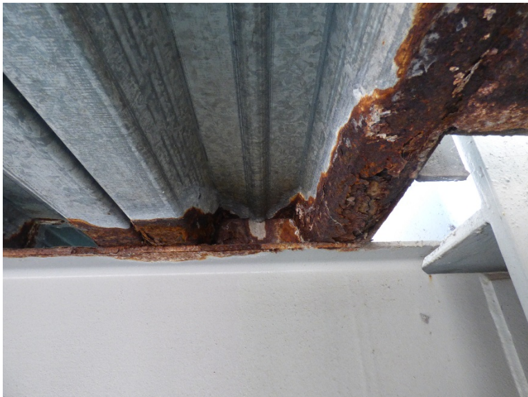
Close up of metal deck damage due to corrosion
