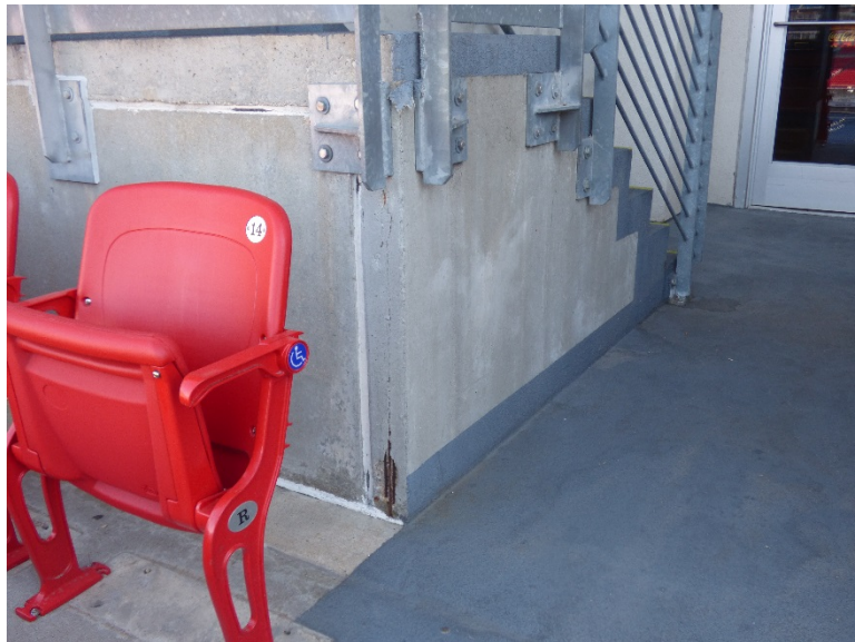
Cracks and spalls at corner of precast stairs
