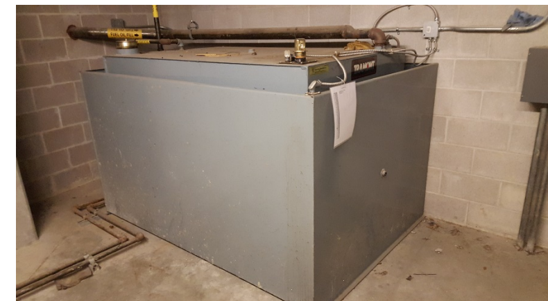
Diesel Generator Day Tank
