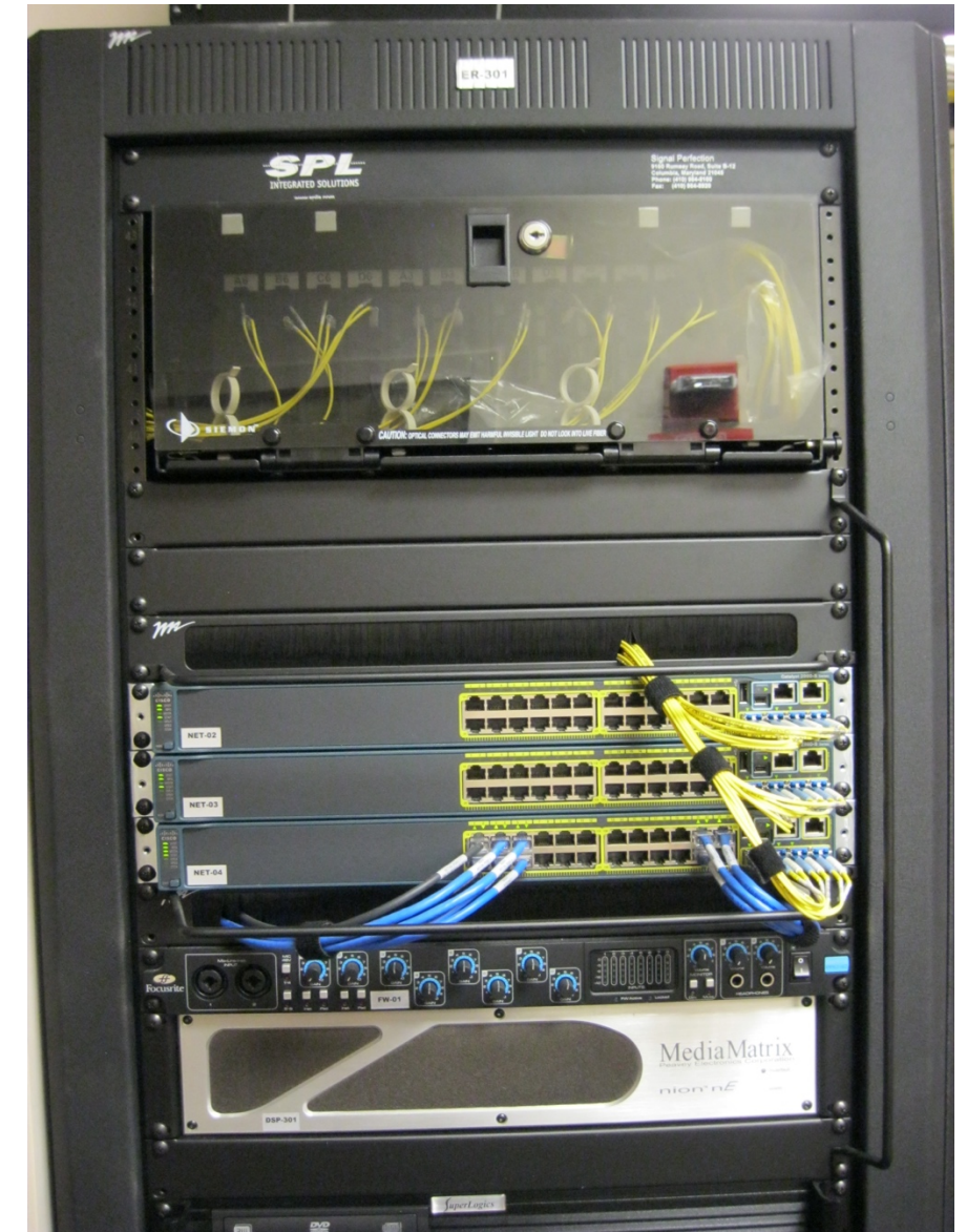
Audio Processor and Amplifier Equipment
