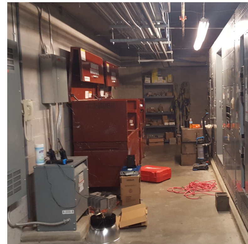
Main Electrical Room Utilized for Storage
