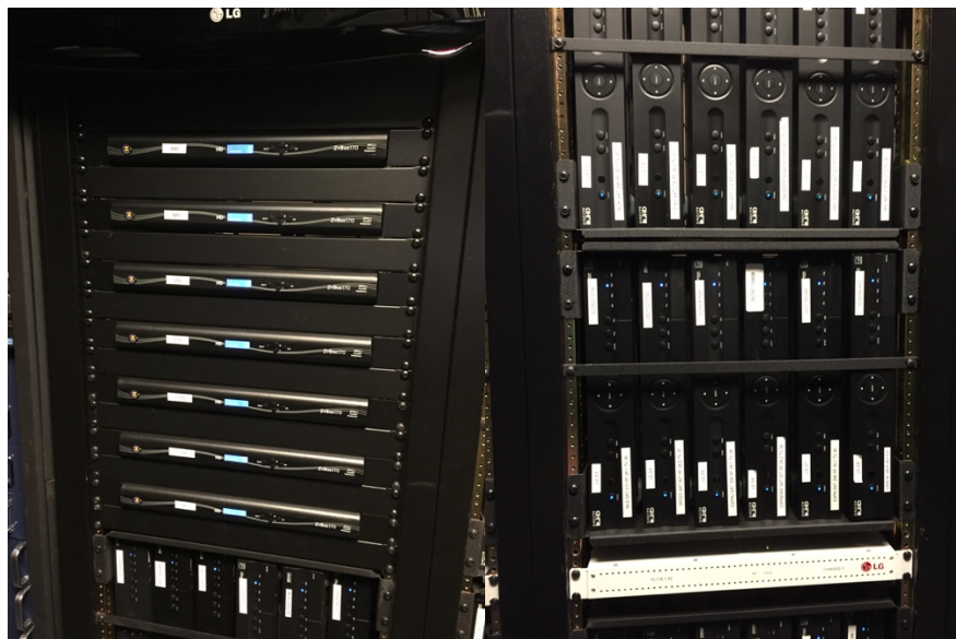
DirecTV Receivers, ZeeVee and LG Encoders
