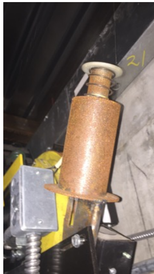
Typical Rusted Governor Equipment Express
