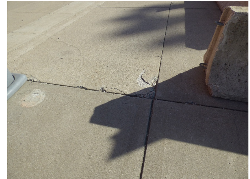
Delaminated concrete in slab-on-grade
