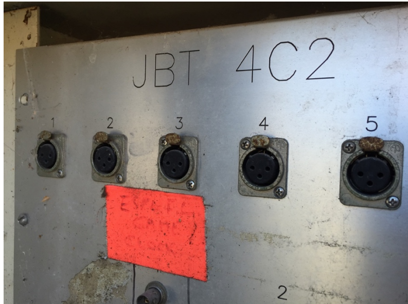
Close Up of Corroded XLR Connectors (Typical of Most)
