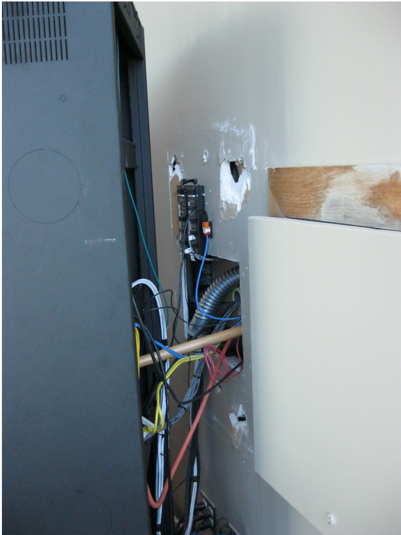
Poor installation workmanship at club AV rack
