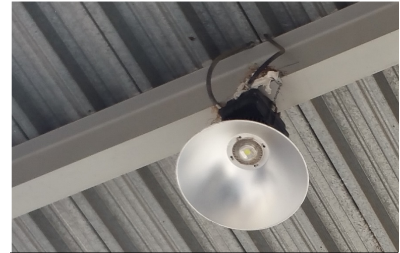
LED High Bay Fixture Located on the Main Concourse
