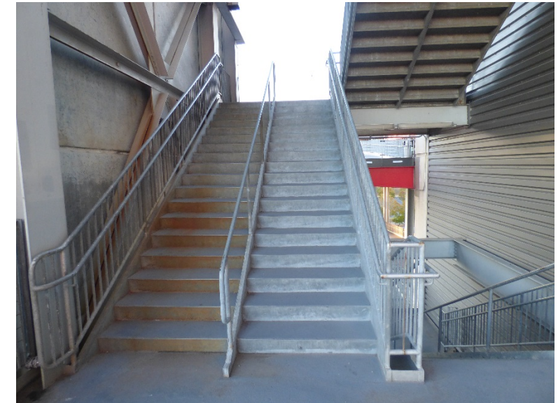
Rust staining of horizontal surfaces below open-ended tubes
