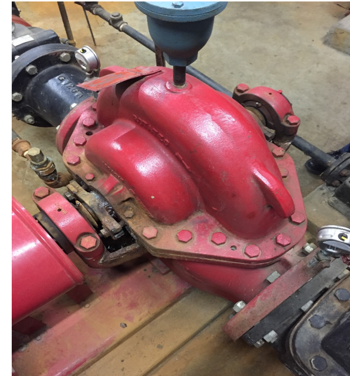
Fire Pump Casing
