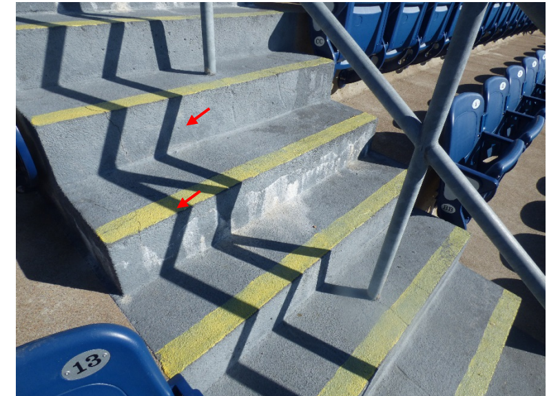
Cracks and leaching in concrete steps
