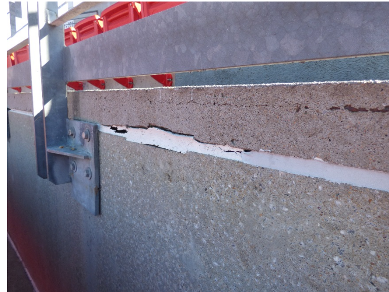
Failed horizontal sealant on precast seating riser
