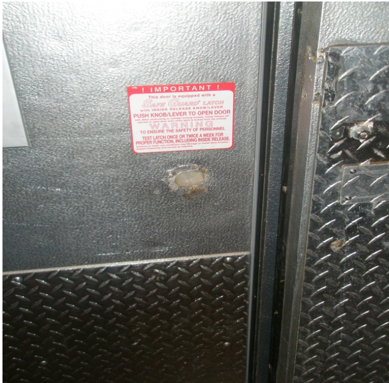
Missing Door hardware on Cooler
