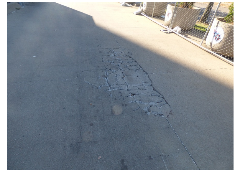
Severely damaged concrete in slab-on-grade
