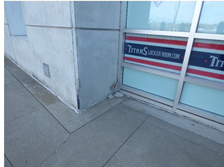
Concrete spall on precast wall element
