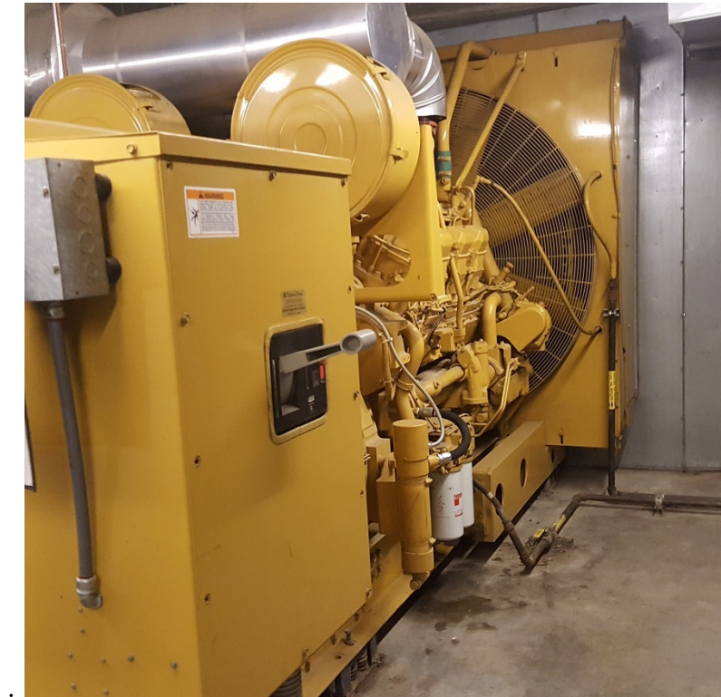
1000 KW Diesel Generator
