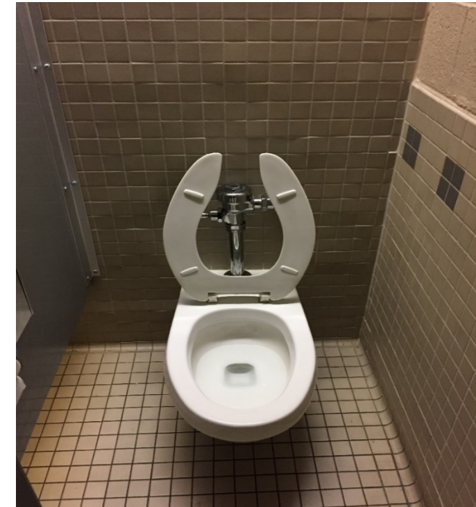
Typical Flush Valve Water Closet
