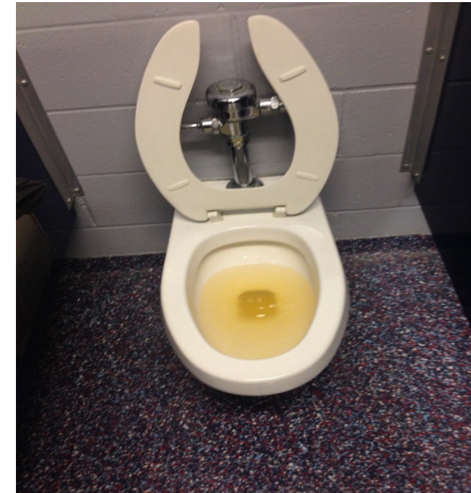
Water Closet Upper Concourse – Discolored Water from Corrosion
