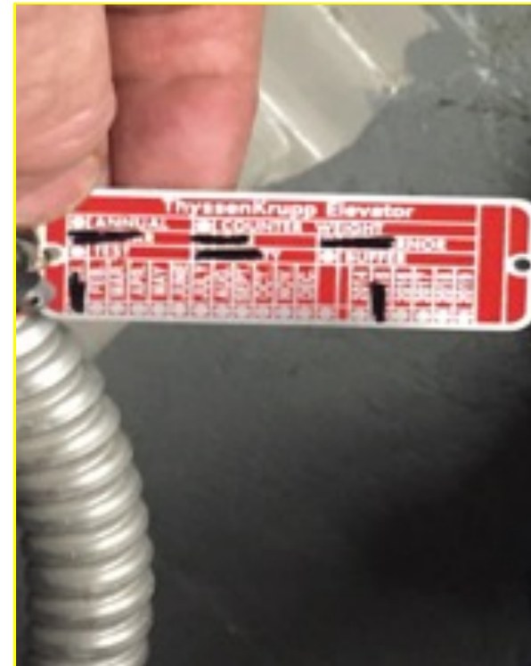
Typical Passenger 5 Year Test Tag
