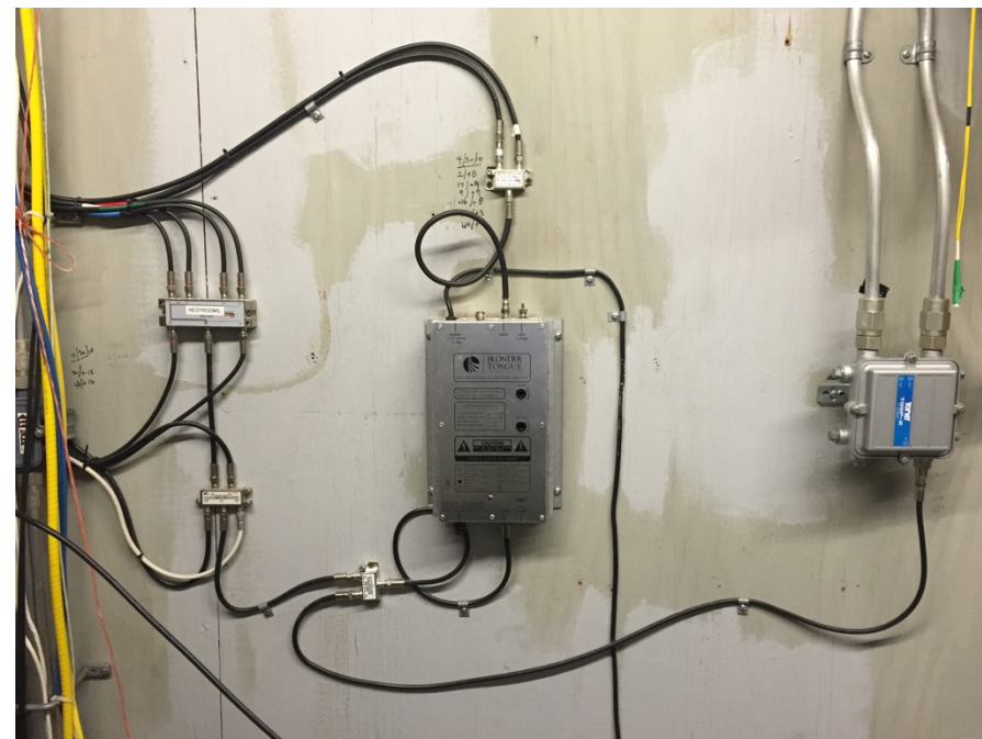
Example of a distribution closet or node
