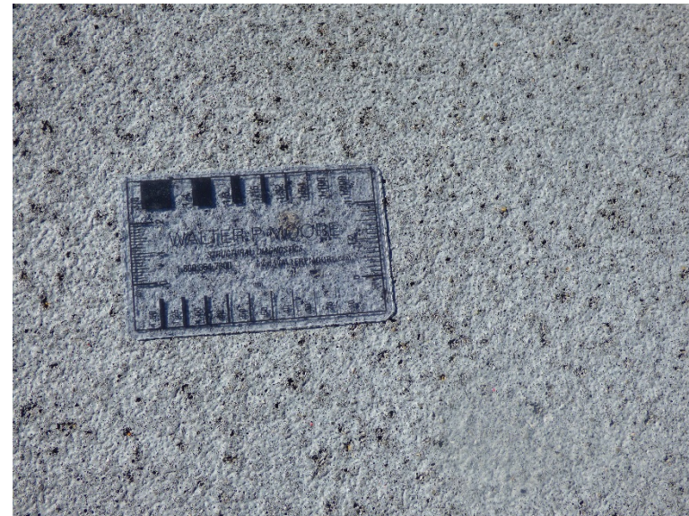
Aged traffic coating on pedestrian ramps
