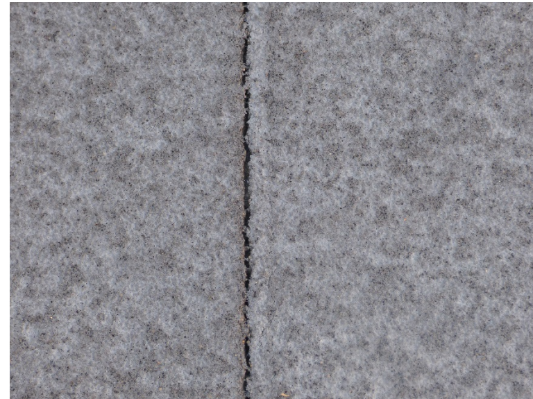
Failed sealant at topping slab joints in the Main Level concourse
