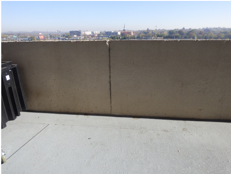
Vertical joint between concrete perimeter walls
