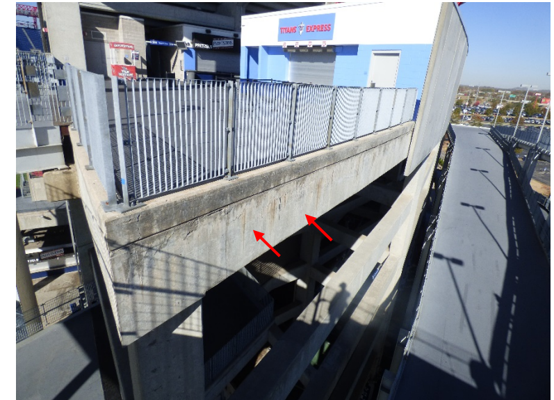
Concrete spalls and delamination on face of beam and slab
