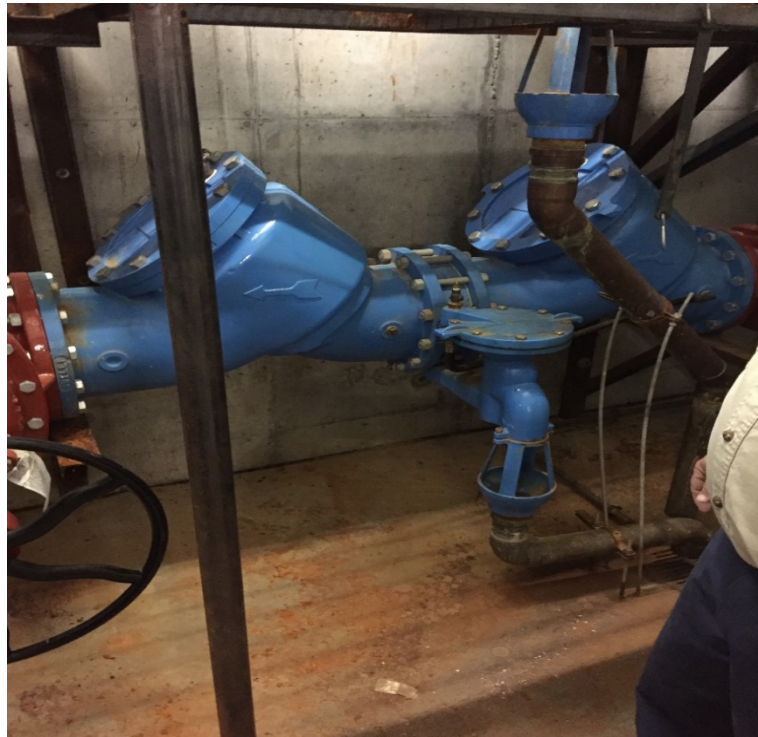
10-inch Reduced Pressure Backflow Preventer on Domestic Water Main
