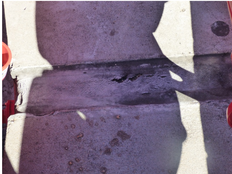
Failed expansion joint on seating areas
