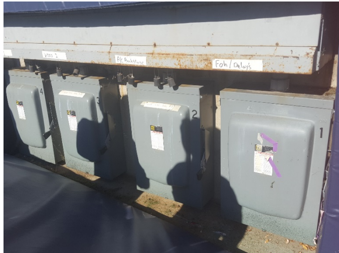
Show Power Disconnect Switches.
