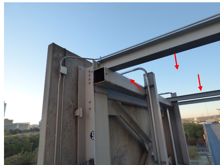
Open ends of steel tubes
