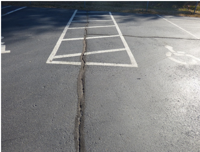
Previously sealed pavement crack
