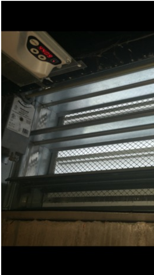
Typical Hoistway Louvered Vent
