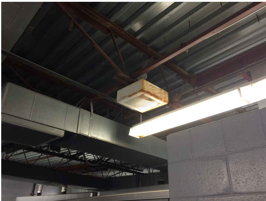
Existing restroom rusted speaker
