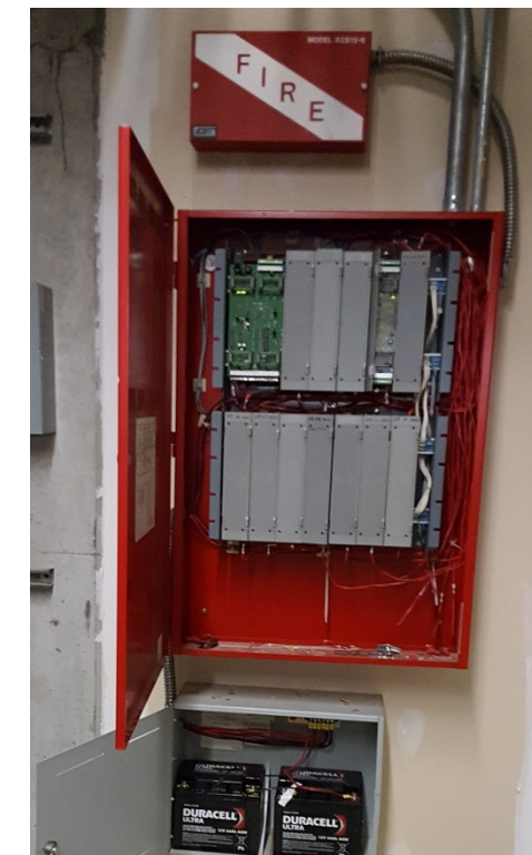
Fire Alarm Riser Panel
