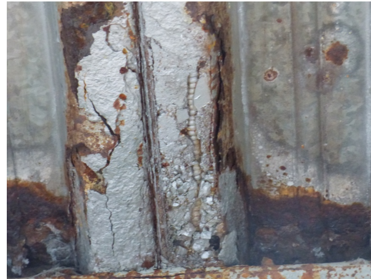
Corroded metal deck which has been painted over at exterior, visible from exterior of stadium sidewalk
