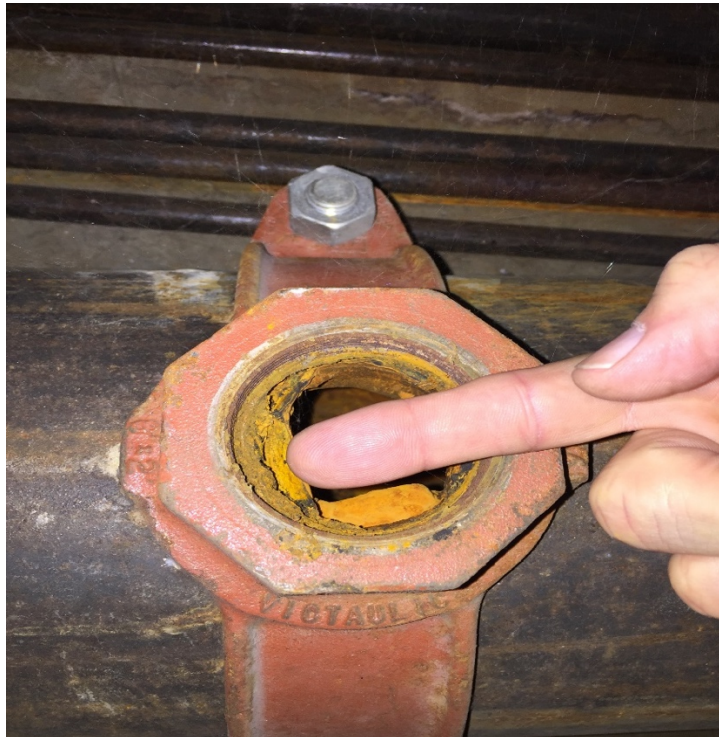
Interior Pipe Corrosion
