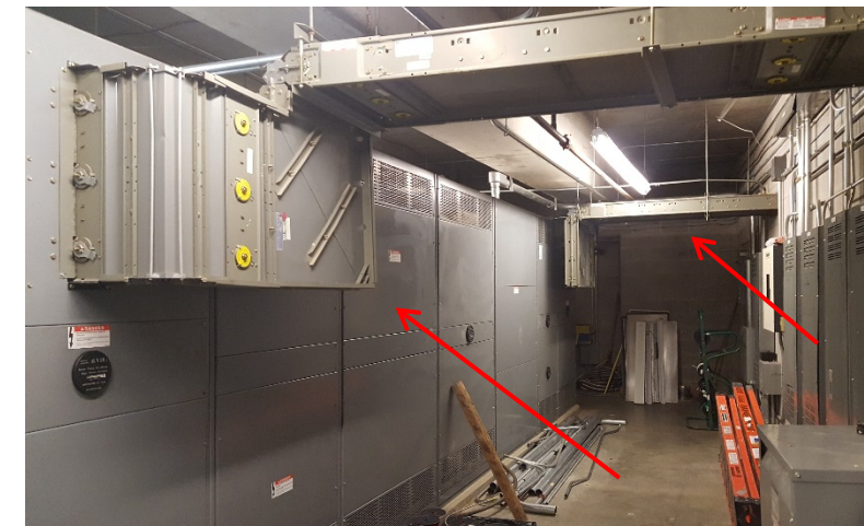
Feeds from NES Vault to Main Switchgear Lineup
