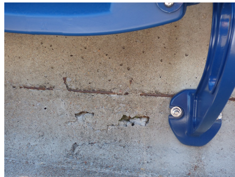
Exposed wire mesh on precast seating riser
