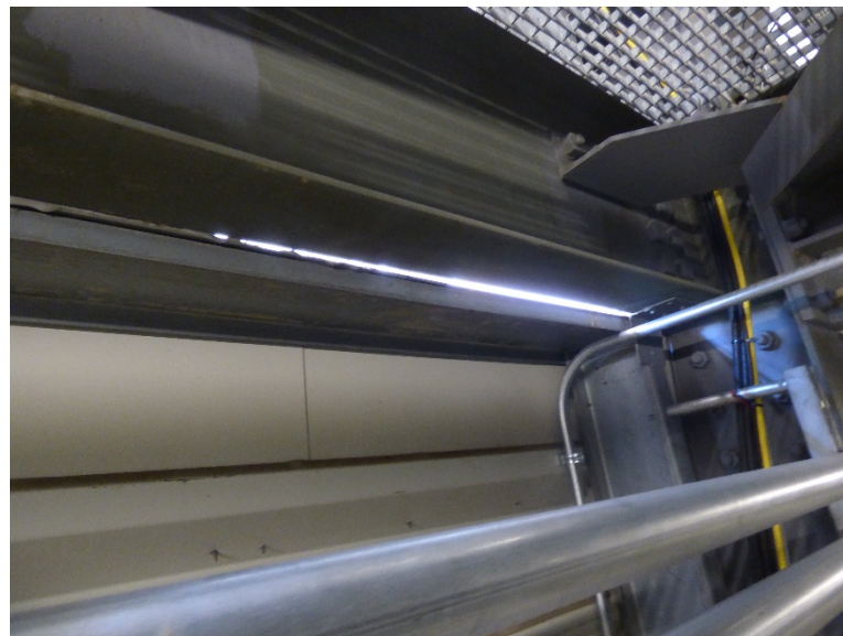
Evidence of failed sealant between elements of scoreboard elements (notice daylight through joint)
