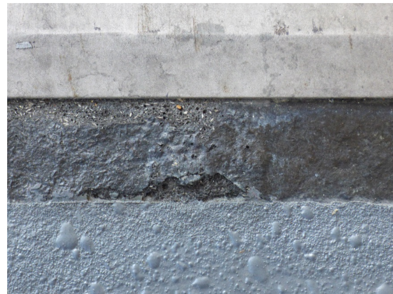
Damage of header material for expansion joint
