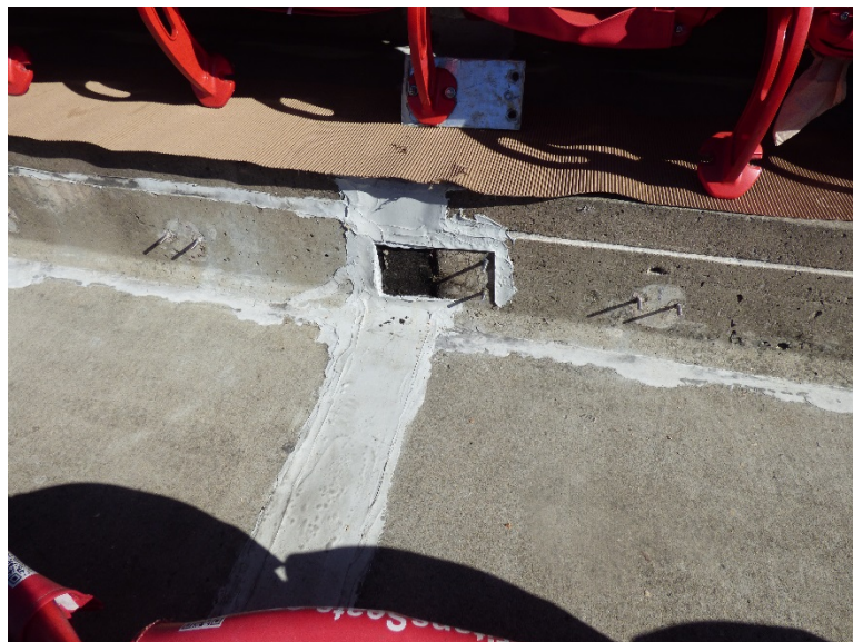
Expansion joint covered with sealant
