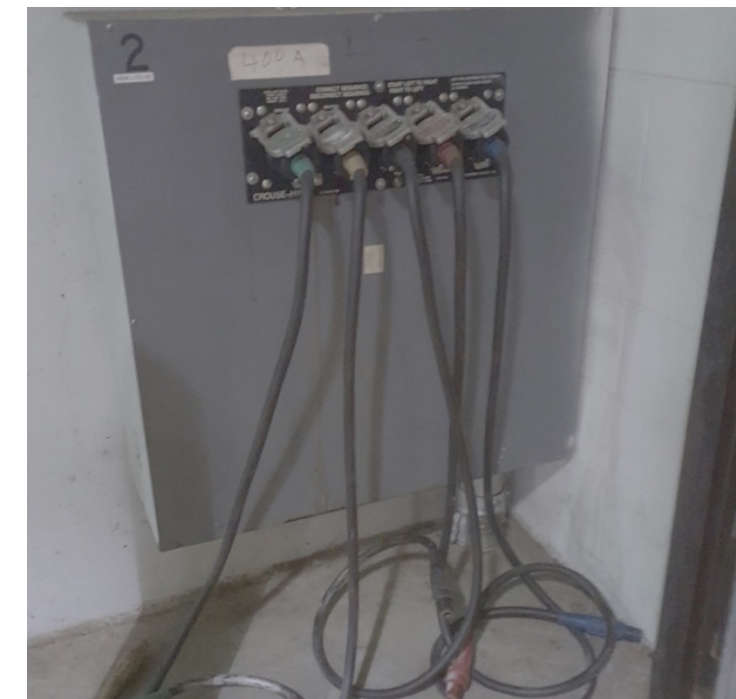
400A Posi-Lok Power Connections
