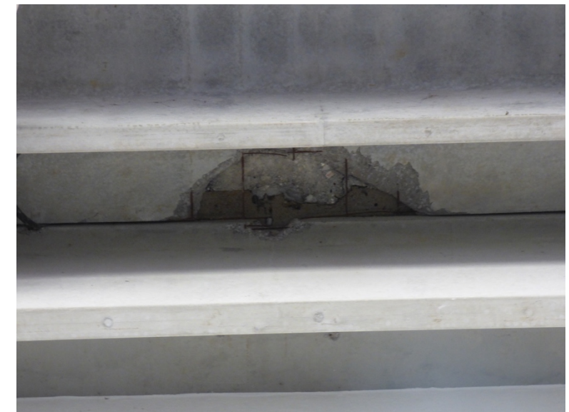
Concrete spall on double-tee flange on the underside of press level, southwest corner of stadium
