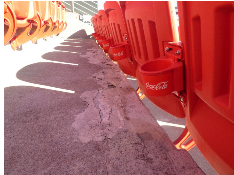
Failed concrete patches on seating risers
