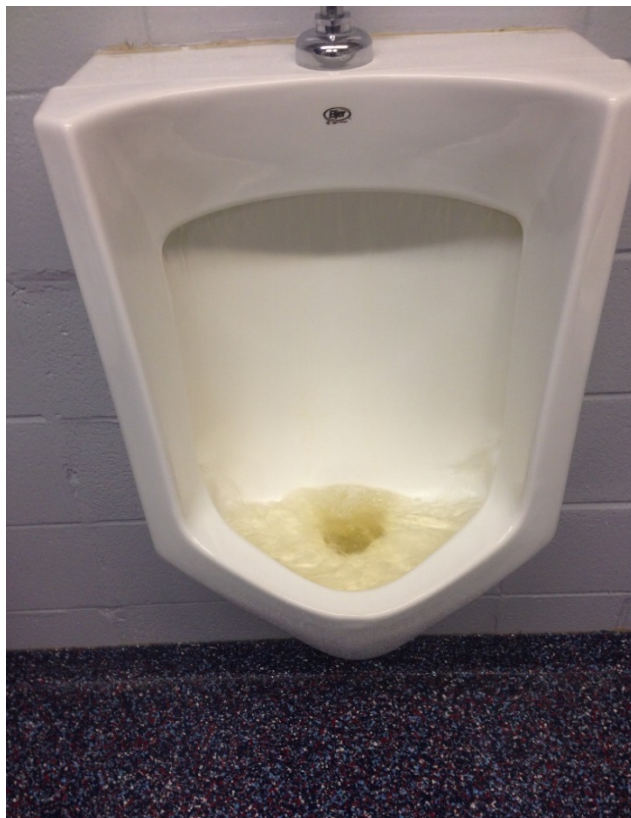
Urinal Upper Concourse – Discolored Water from Corrosion
