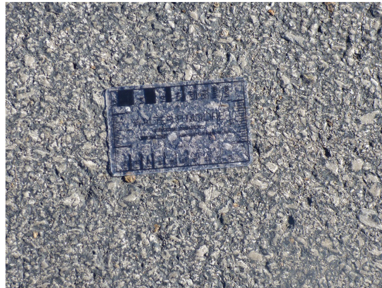
Weathering of pavement
