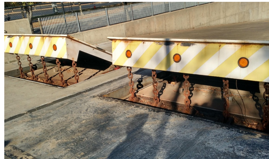
K12 Vehicle Barrier – Loading Dock Truck Entrance
