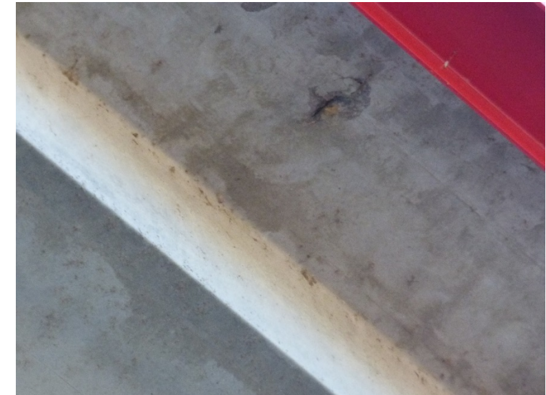
Concrete spall on underside of seating riser.
