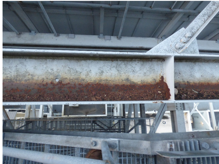
Corrosion of web on structural steel beam. View looking down.
