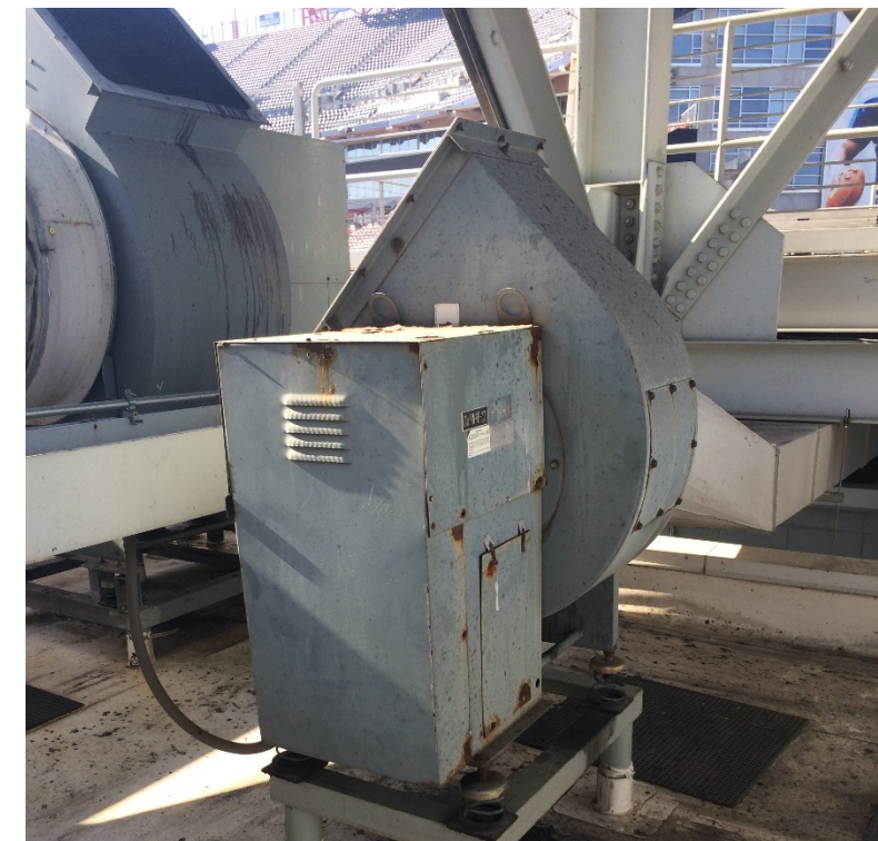
Grease Fan on Low Roof
