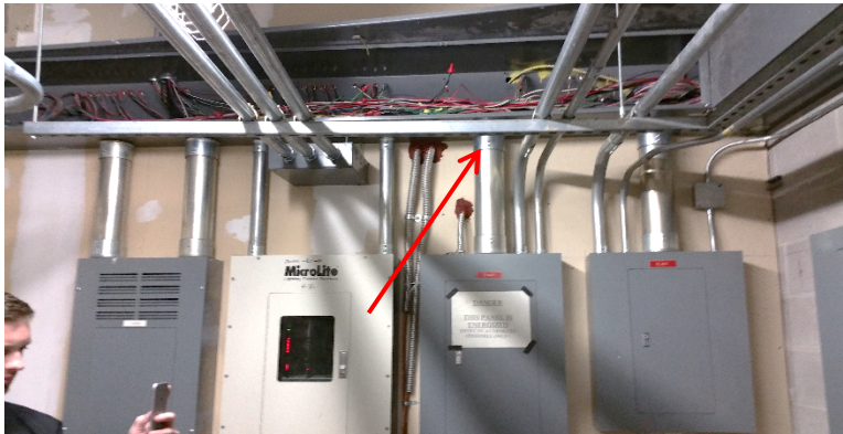
Normal and Emergency Circuits run in the same wireway which is missing the cover
