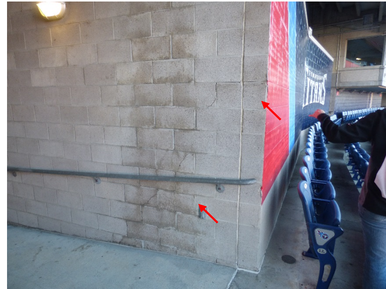
Cracks in concrete masonry units (CMU)
