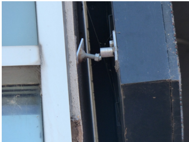
Loose connection of ribbon board
