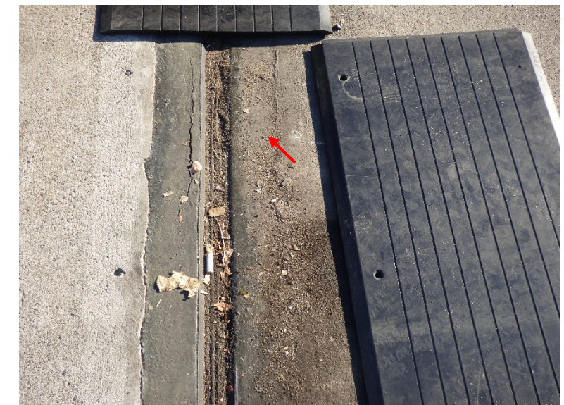
Damage to header material on exterior expansion joint over loading dock
