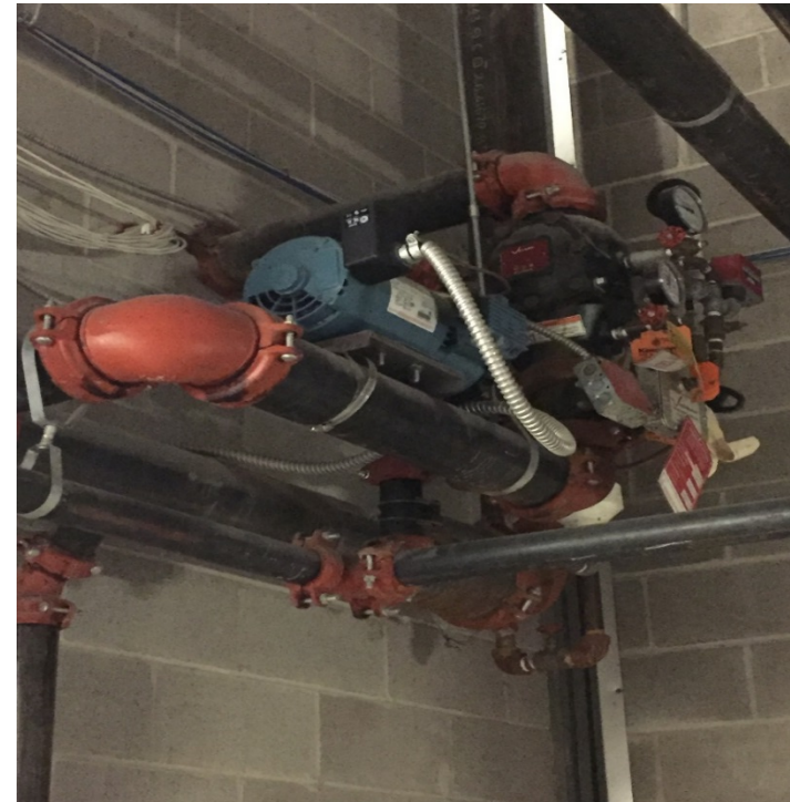
Dry Pipe Valve Assembly and Air Compressor In Stairwell serving Upper Concourse Concessions
