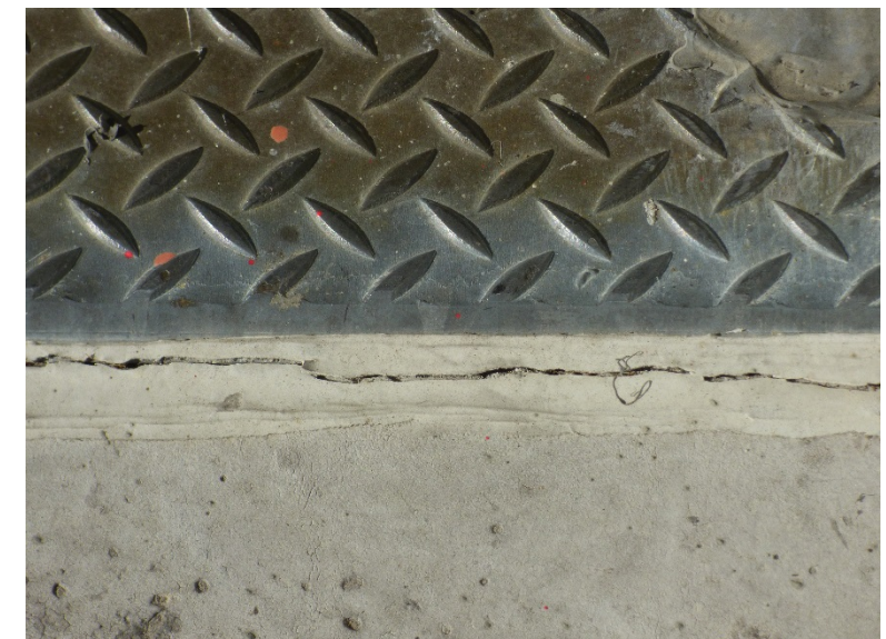
Failed sealant on perimeter of plates over older expansion joints
