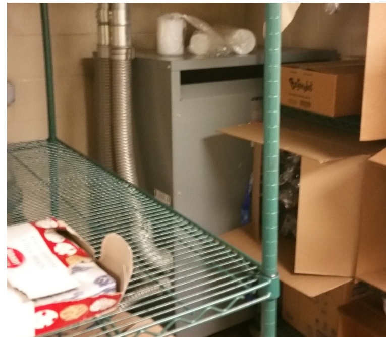
Concession Transformer with Improper Clearance
