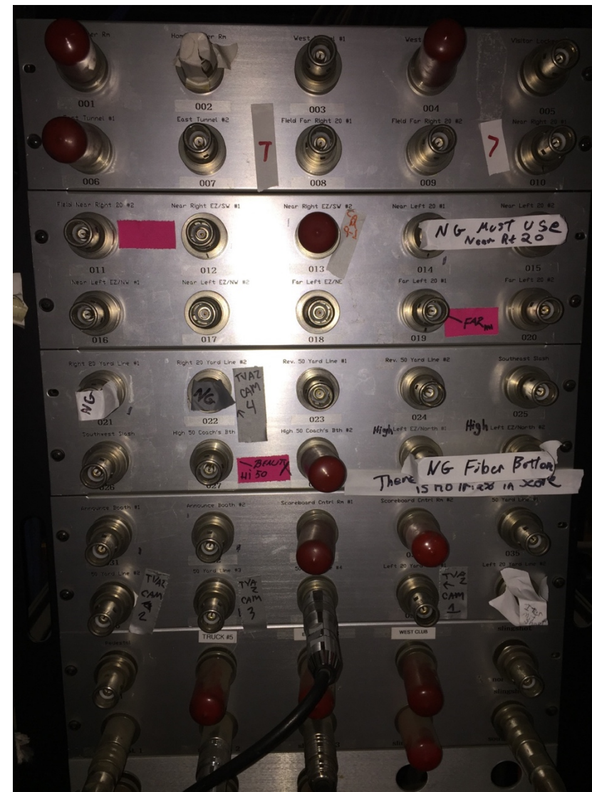
TV Truck Connection Triax Panel
