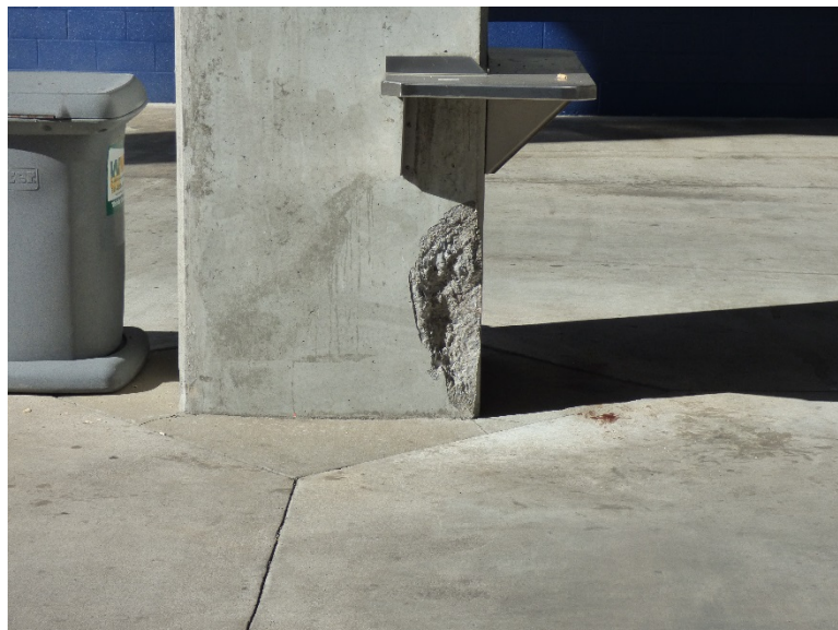
Concrete spall on column at Gridline 10 on main concourse level
