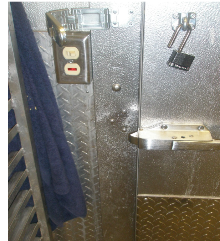
Door Handle on Walk In Cooler is Damaged
