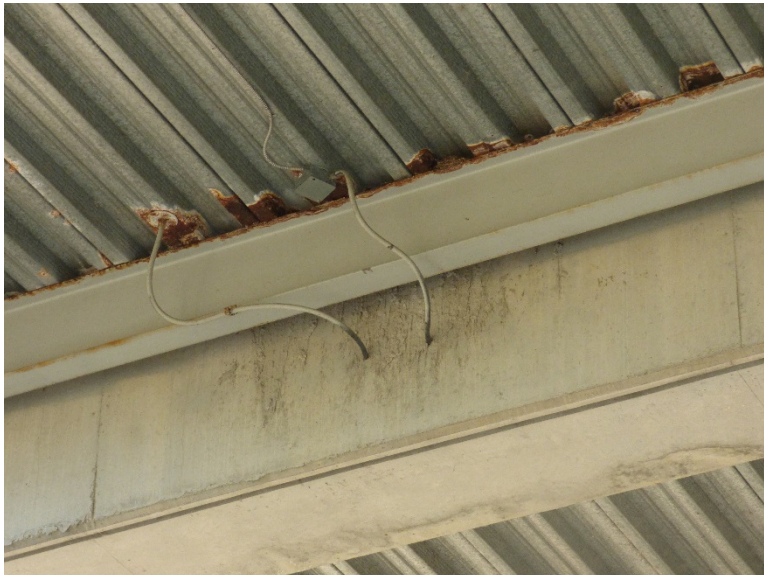
Corrosion of metal deck on pedestrian ramp
