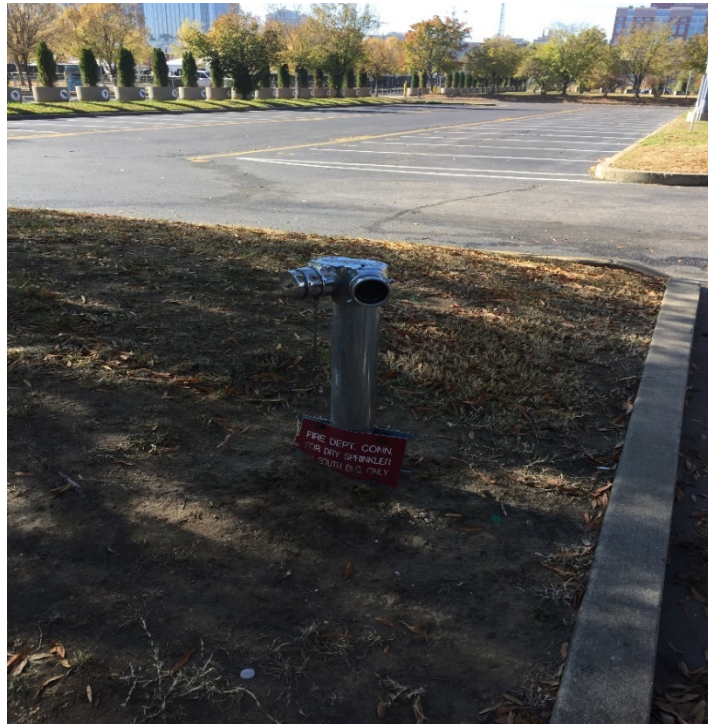
Fire Department Connection South End Zone Missing Caps and Chains
