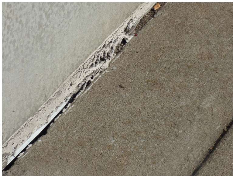
Failed cove sealant at exterior wall
