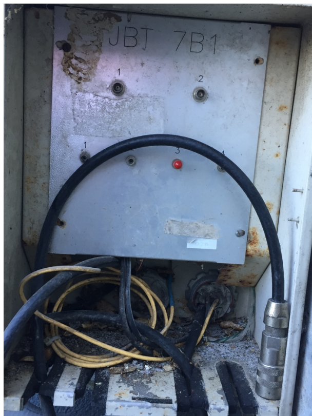
Close Up of Corroded Coax and Fiber Connectors and non-panel terminated triax.
