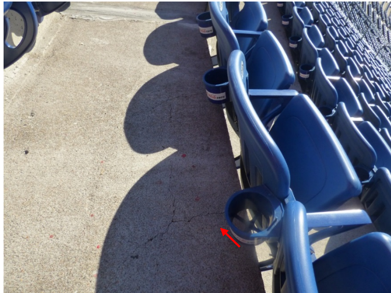
Cracks on seating risers
