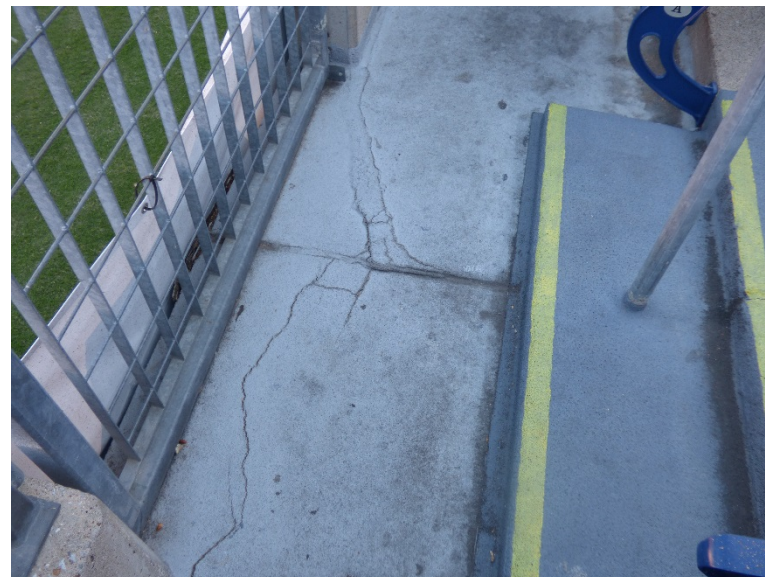
Concrete delaminations on first row of lower level seating area
