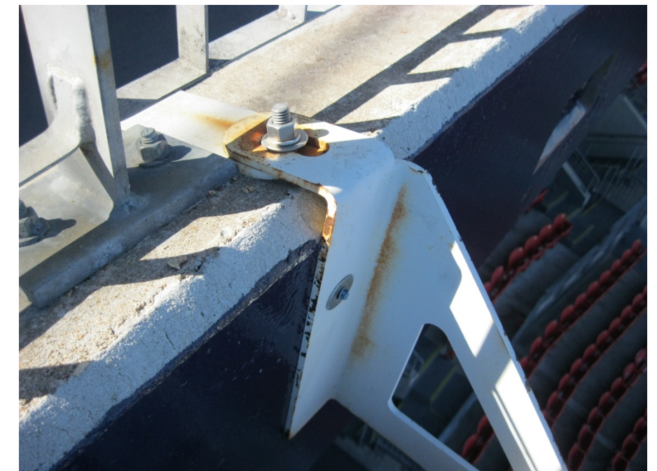
Existing speaker bracket showing rust
