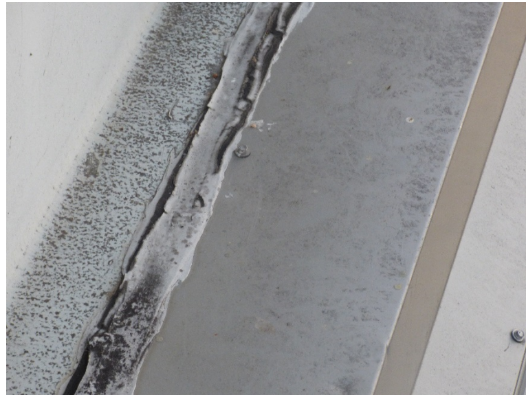
Deteriorated sealant at joint on scoreboard elements
