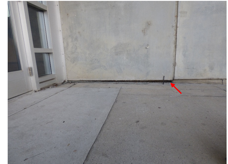
Missing grout below exterior precast wall panel
