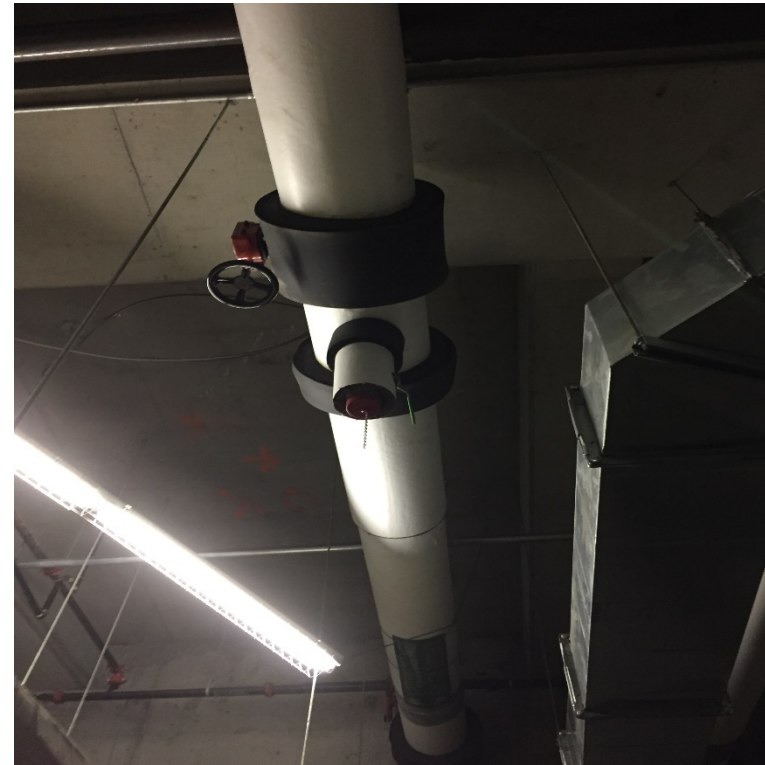
Domestic Water Drainage Port – Event Level
