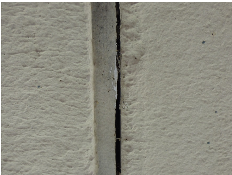
Failed sealant at joint between perimeter walls
