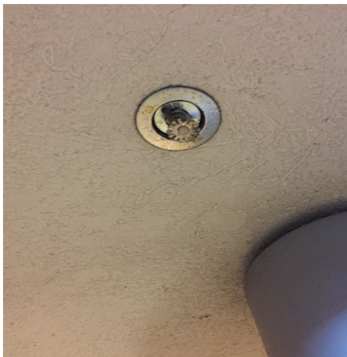
Automatic Sprinkler Head Corrosion
