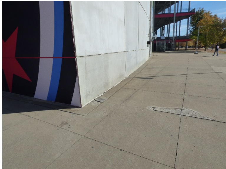
View of exterior wall location of failed cove sealant
