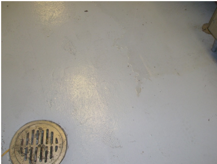
Floor slopes away from floor drain in concession stand
