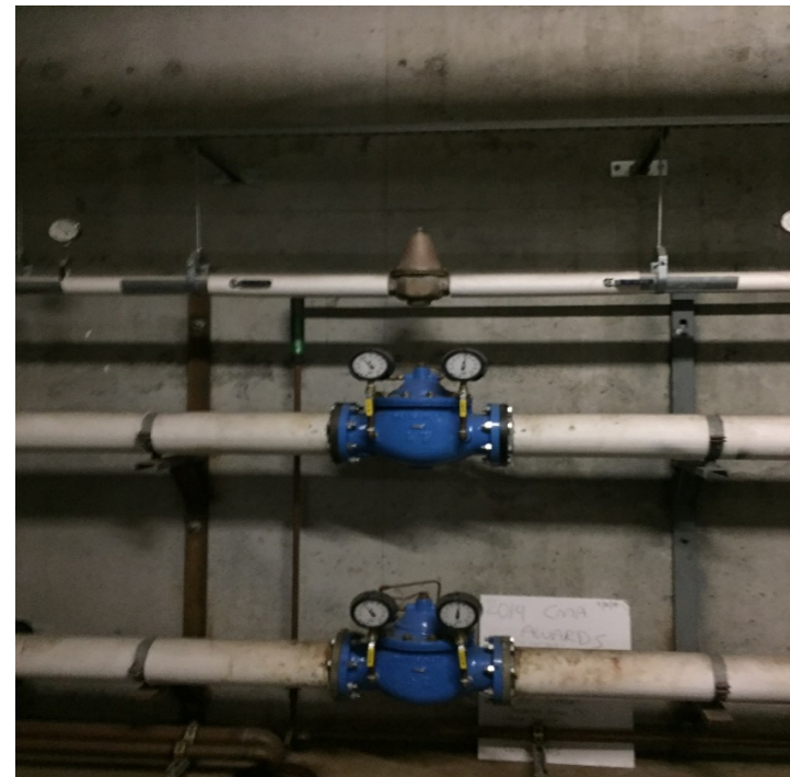
Building Pressure Reducing Valve Station
