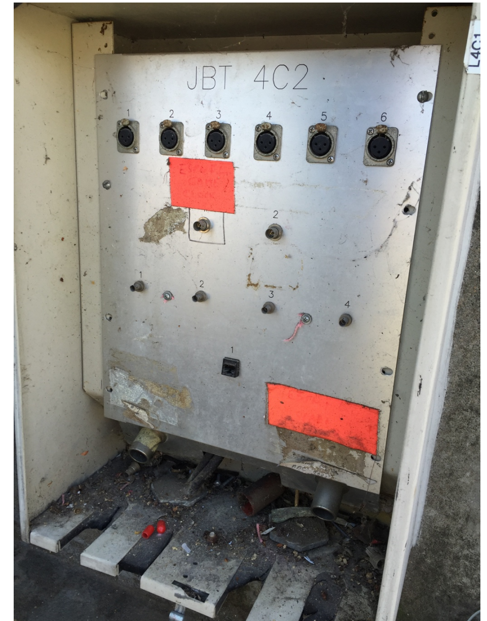
Damaged and Corroded Broadcast Box Panel (Typical of most)
