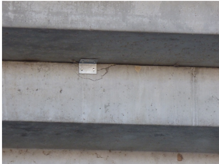
Concrete delamination at clip angle location
