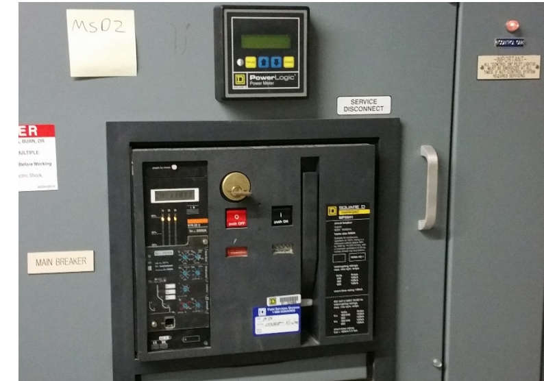
Main Breaker and Analog Meter
