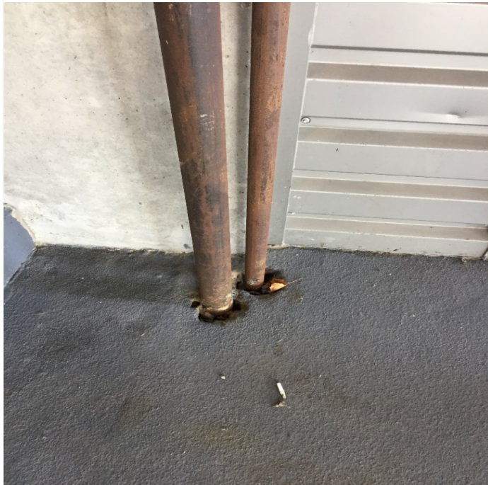
Piping Missing Floor Supports
