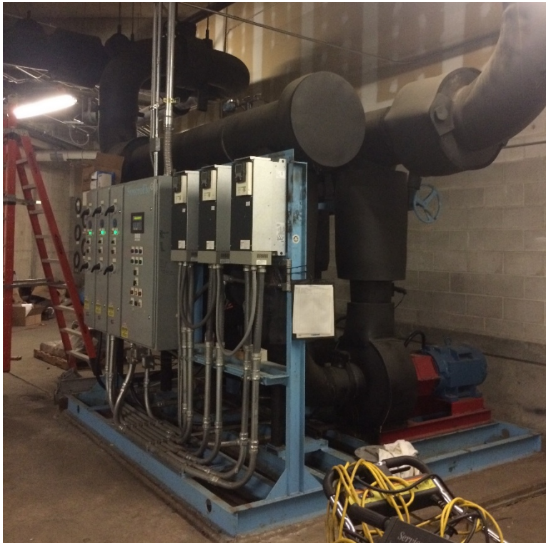
Primary Chilled Water Pump Skid
