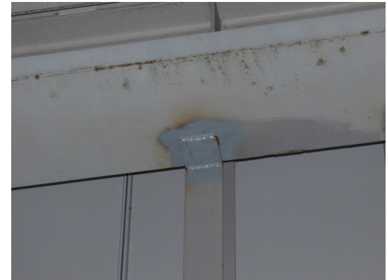
Evidence of rust on previously coated clip angle
