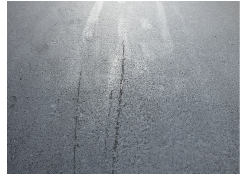
Damaged traffic coating on ramp
