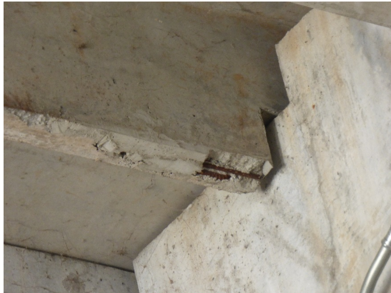
Concrete spall on double-tee stem
