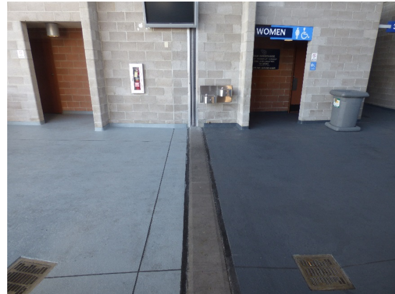
Overall view of new expansion joint on upper concourse
