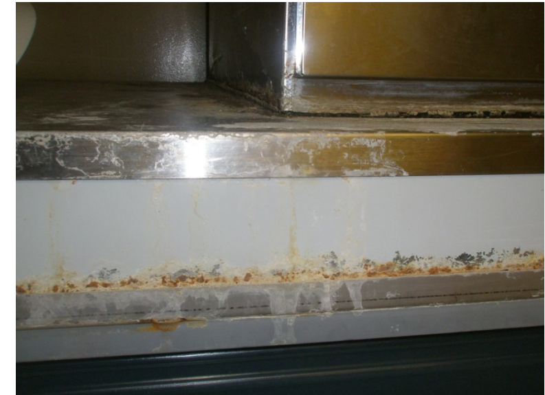
Mineral Build Up on Ice Machine
