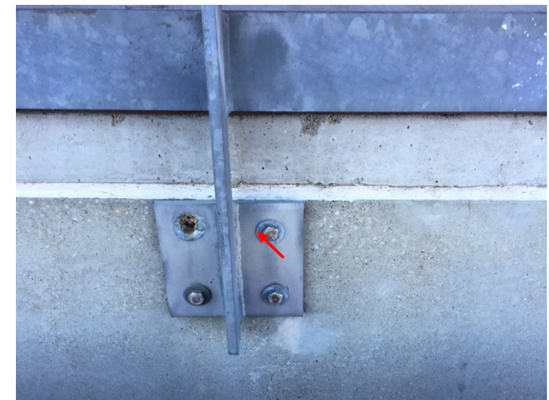
Missing bolt on handrail anchorage plate in club level
