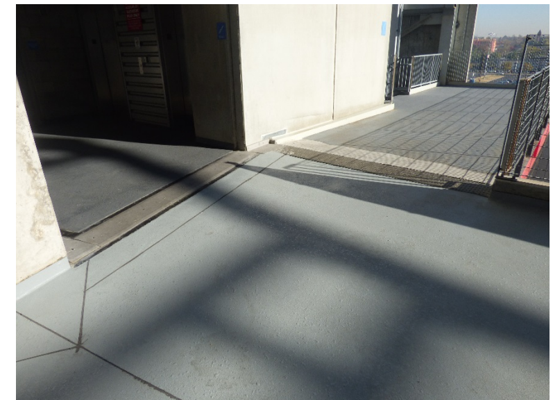
Overview of older expansion joints
