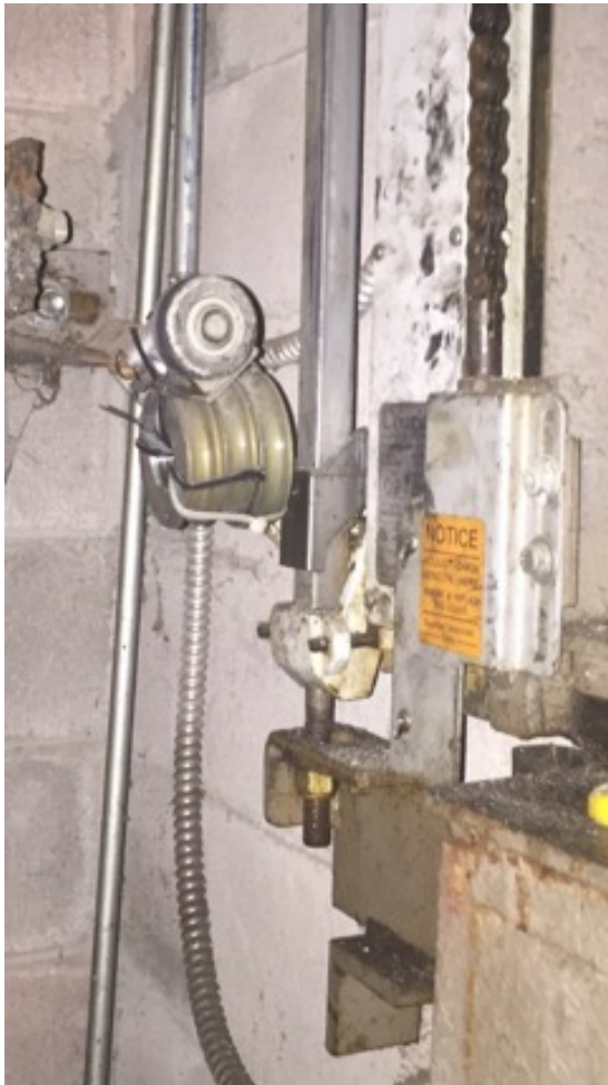
Field Engineered Gate Switch in need of Repair
