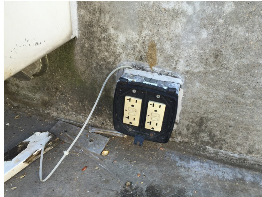
Non-weatherized outlet subject to standing water
