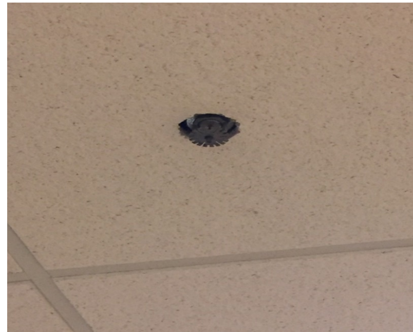
Interior Automatic Sprinkler Head Missing Trim
