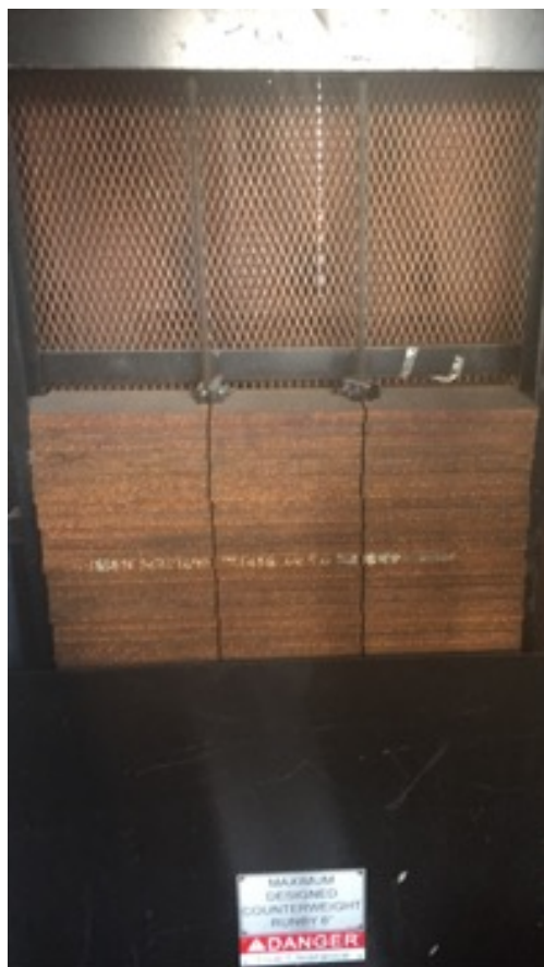
Typical Rusted Counterweights on Express Cars
