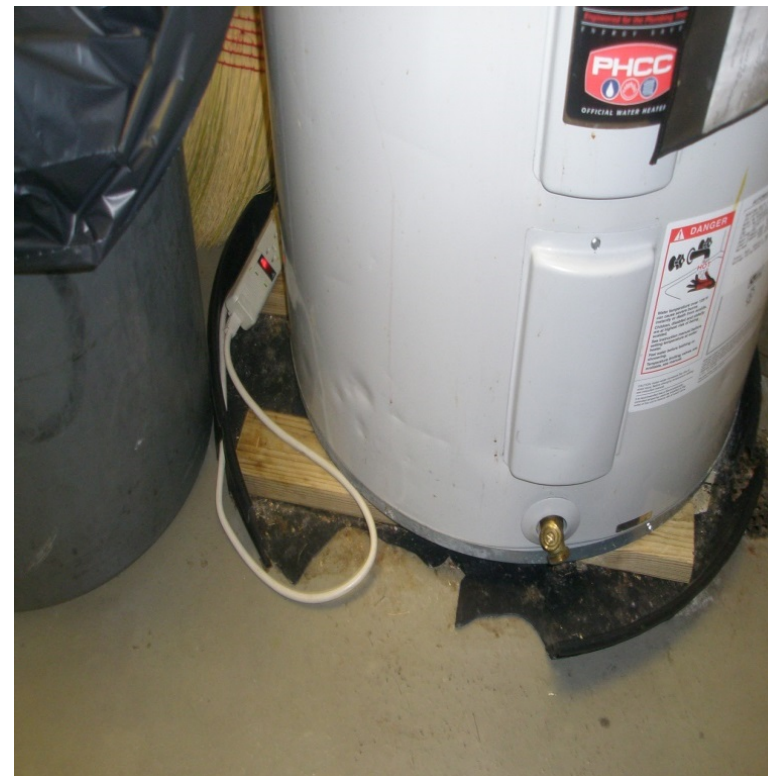
Non-code compliant stand for hot water heater
