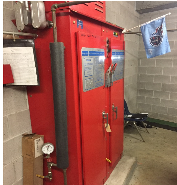
Fire Pump Controller
