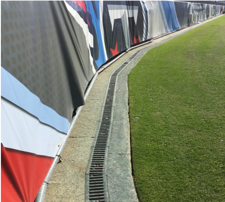
Playing Field Trench Drain
