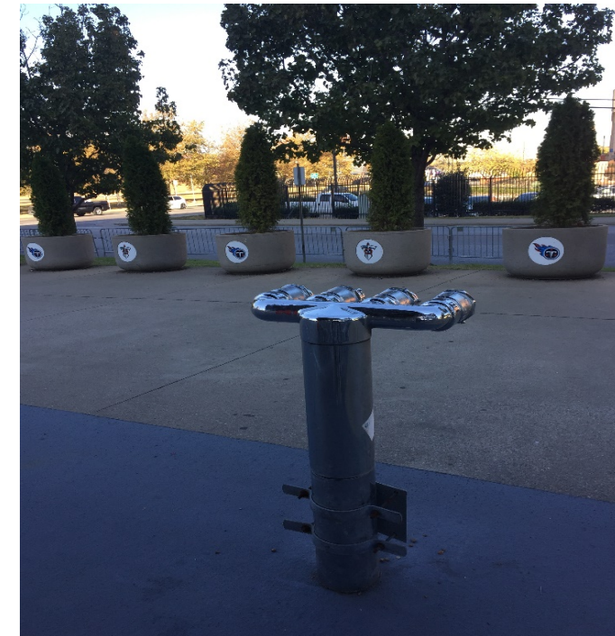
Fire Department Connection West, North and East Sides Missing Caps and Chains
