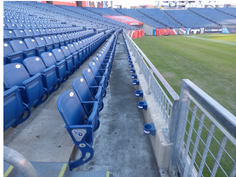
Deteriorated traffic coating
