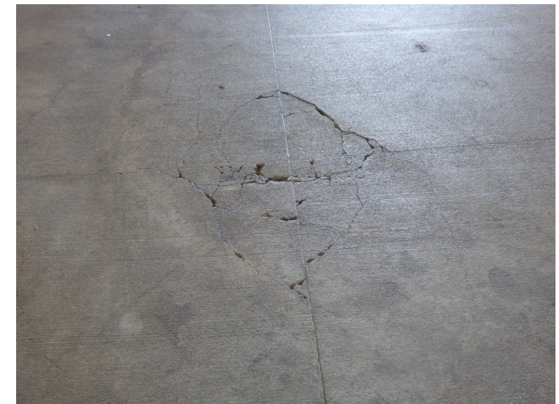
Concrete spalls on slab-on-grade
