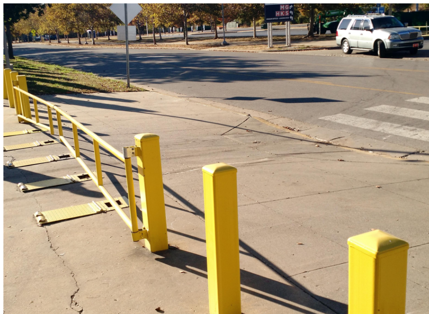
Physical Security Barriers – Removable Bollards and Gates
