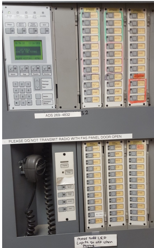
Fire Alarm Control Panel
