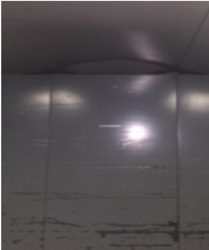
Damaged Interior Ceiling on Freight #4
