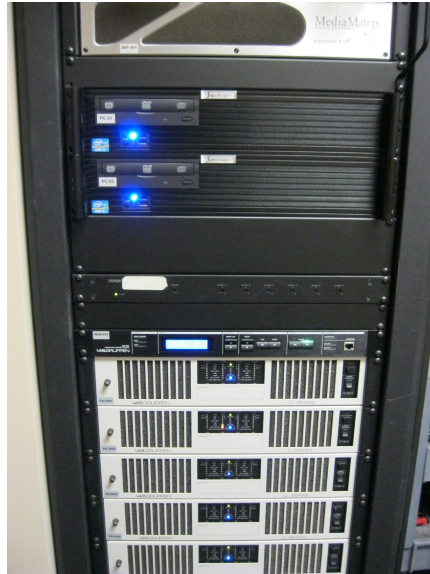
Audio Processor and Amplifier Equipment
