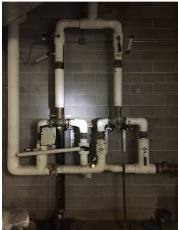
Holby Mixing Valve Station
