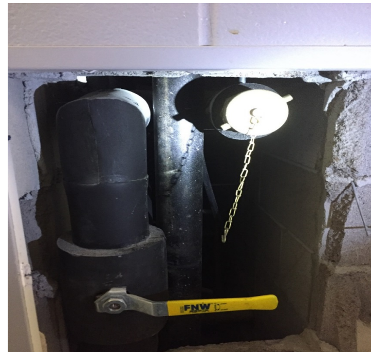
Domestic Water Flushing Port – Upper Concourse
