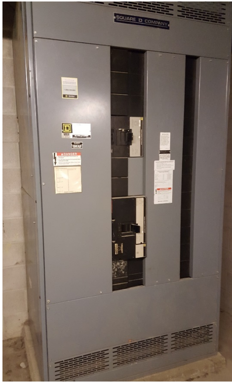
Generator Distribution Board
