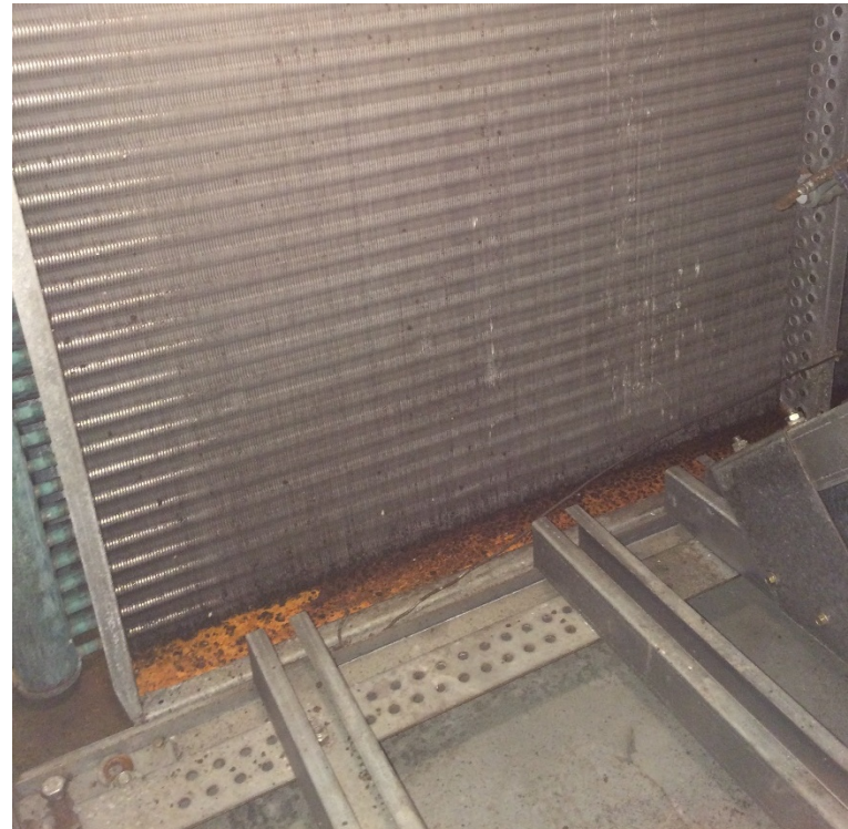
Air Handling Cooling Coil with Biological Growth
