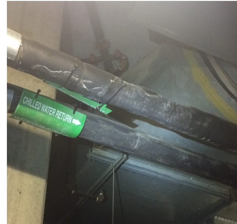
Chilled Water Insulation
