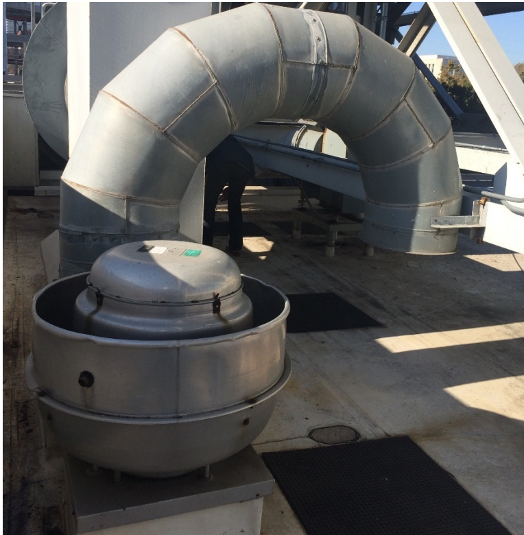
General Exhaust Fan on Low Roof
