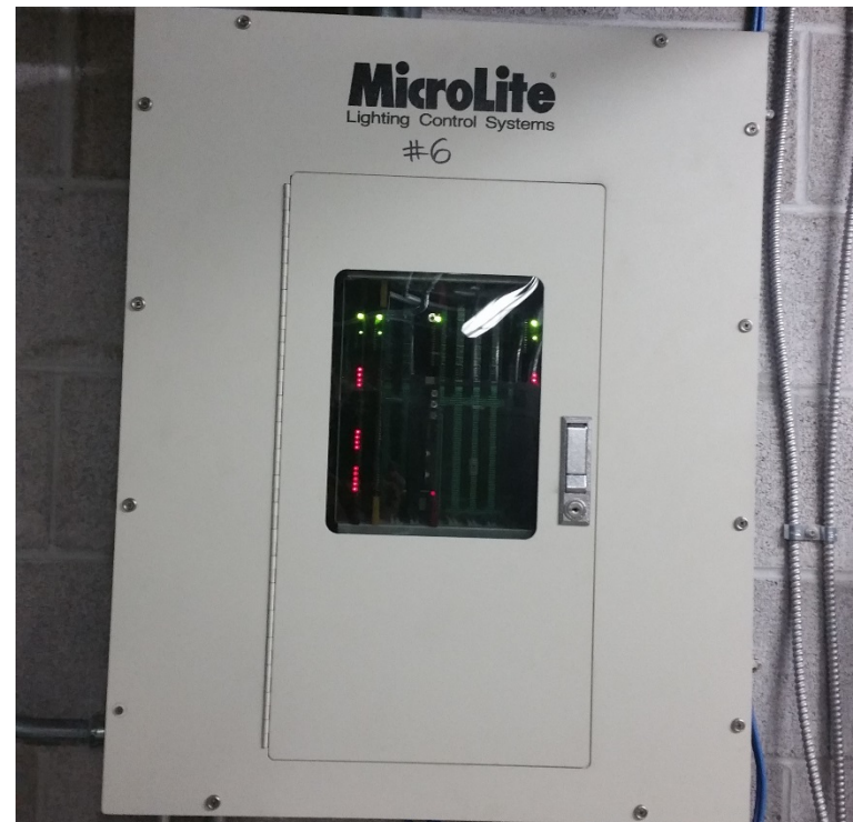
Existing MicroLite Relay Panel
