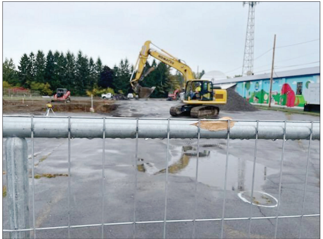
Construction at the new 7Brew drive-up stand on Arsenal Street began Tuesday. It should take just a few months to get the 510-square-foot stand coffee stand up and running. Craig Fox/Watertown Daily Times
