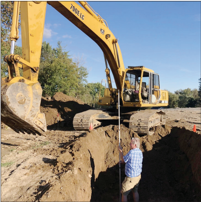
Gary Johnson dug the first hole to start the project, prepping for the first canopy, on Sept. 24, 2022. Photo by Jessica Johnson
