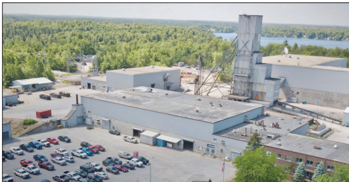
Empire State Mines LLC plans to eventually employ 55 additional full-time equivalent employees and support the retention of 135 current employees if it is approved for $1 million in funding from the New York Power Authority. Watertown Daily Times
