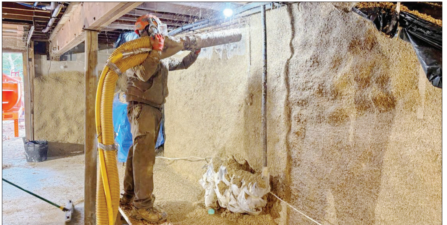
Builder Jeff Gagnon uses the Eready spray system - recently purchased by Cornell for community use - to insulate a basement in Ulster County with hemp lime, a composite of hemp hurd and lime binder. Photo courtesy of Build Green Now
