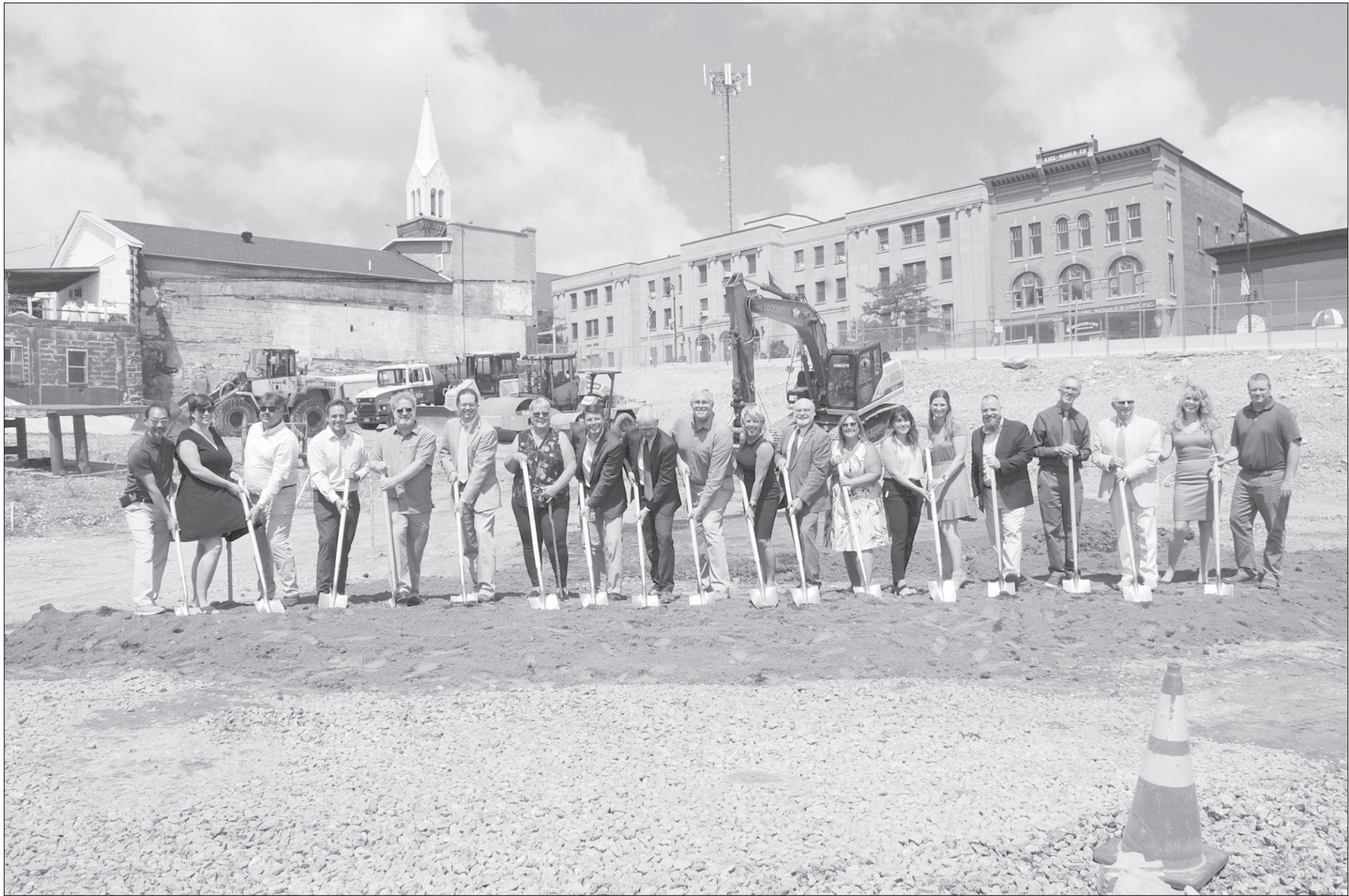
Officials gathered for the official groundbreaking on the Harison Place Project in Malone in July. Pictured, from left, are Felix Tam, Citizen Advocates Foundation board chair; Deanna Smith, Citizen Advocates board chair; Sam Celia, Celia Construction; Dave Harris, NBT Bank; Tony Thesing, National Equity Fund; Darren Scott, Upstate East Director of Development, Homes and Community Renewal; Andrea Stewart, Malone town supervisor; Assemblymember Billy Jones (D-Chateaugay); James Button, Citizen Advocates, Inc. president and chief executive officer; state Senator Daniel G. Stec (R-Queensbury); Malone Mayor Andrea Dumas; Franklin County Legislator Donald Dabiew (D-Bombay); Dana Greenberg, Office of Temporary and Disability Assistance; Isabel Bazaldua, Office of Mental Health; Stephen Hunt, Empire State Development; Bruce Levine, 3d Development; Paul Goodrow, Harison Place board chair; Lindsay Hendricks, 3d Development; Nick Eells, Citizen Advocates board member. Trevor Buchanan/Malone Telegram
