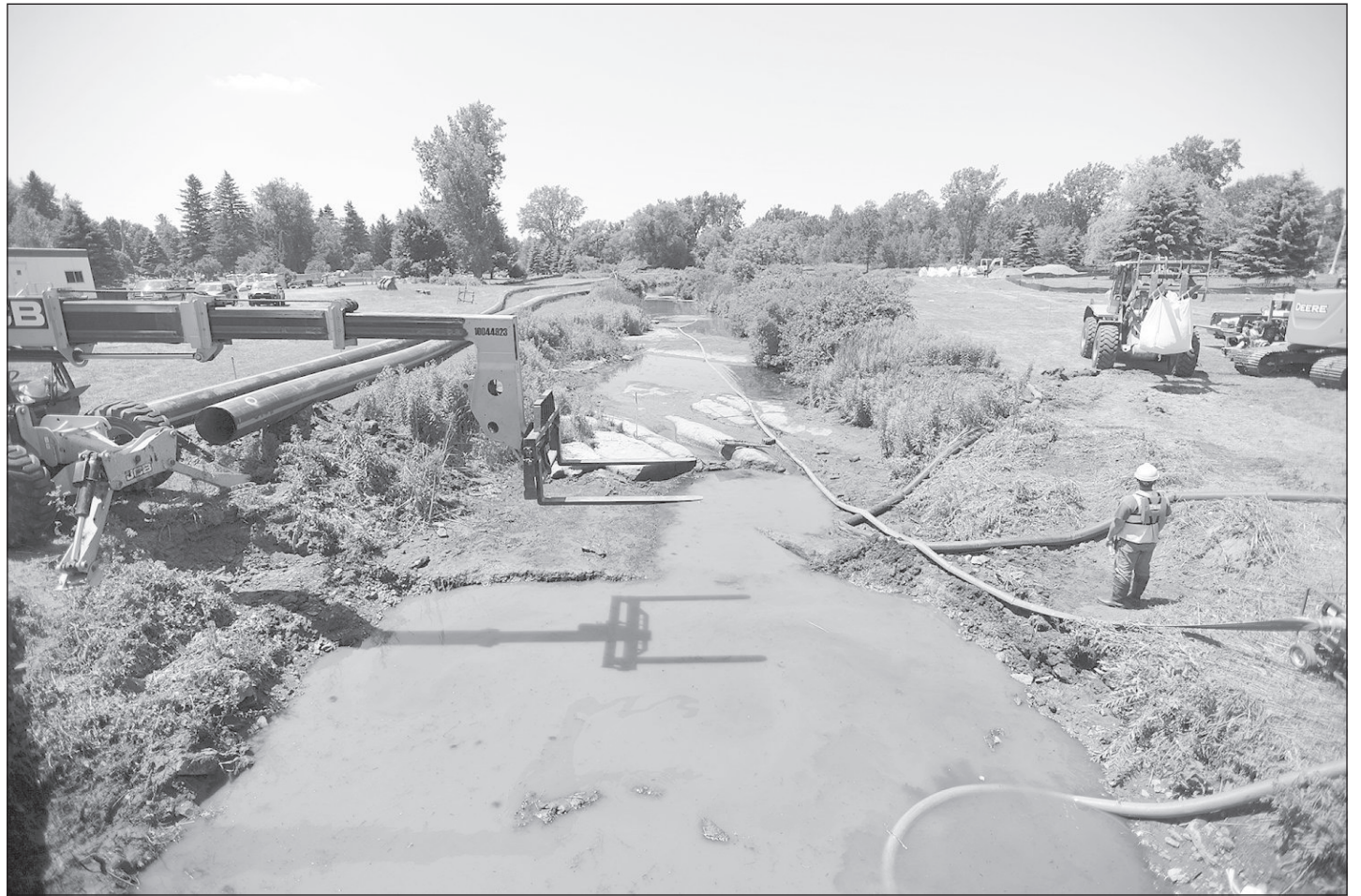
Construction crews work on a water diversion project on Kelsey Creek in Watertown in 2016. Watertown Daily Times
