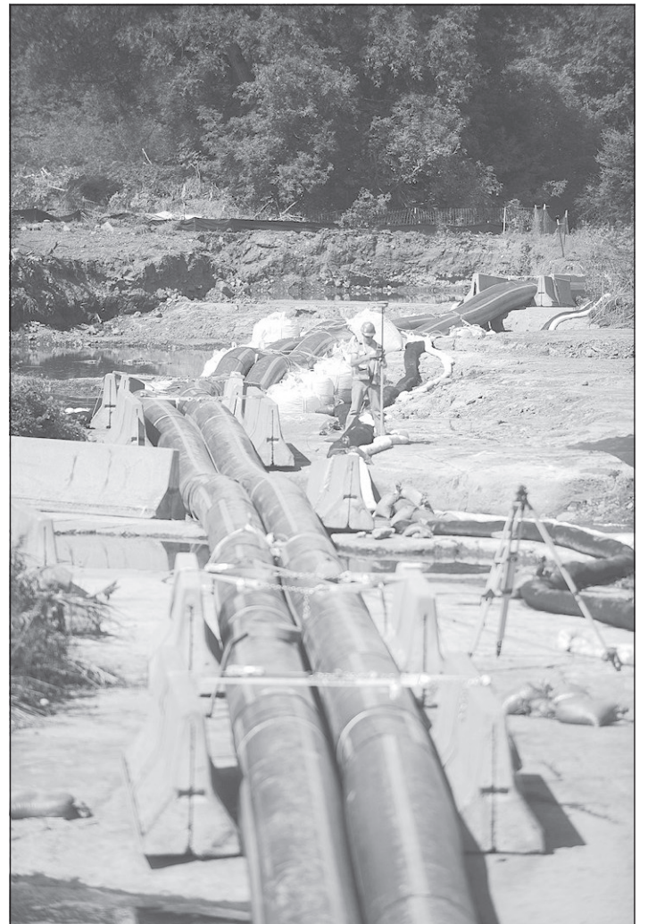
Construction crews work on a water diversion project on Kelsey Creek in Watertown in 2016. Watertown Daily Times
