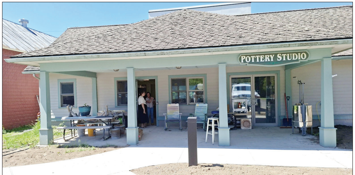
Left: The pottery studio, part of the expanded campus of the Thousand Islands Arts Center, will soon be getting a new roof.
