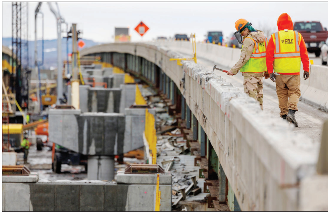
Interstate 481 at Kirkville Road and the CSX rail yard in DeWitt is widened in February 2025 as part of the Interstate 81 project. N. Scott Trimble/syracuse.com/TNS
