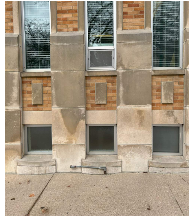
WALKS POURED TO LIMESTONE BASE
