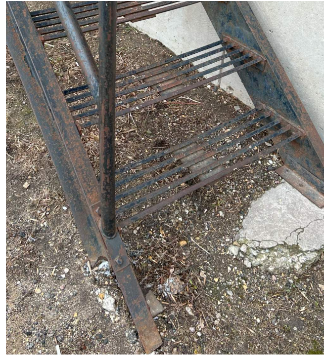
BASE OF EGRESS STAIR
