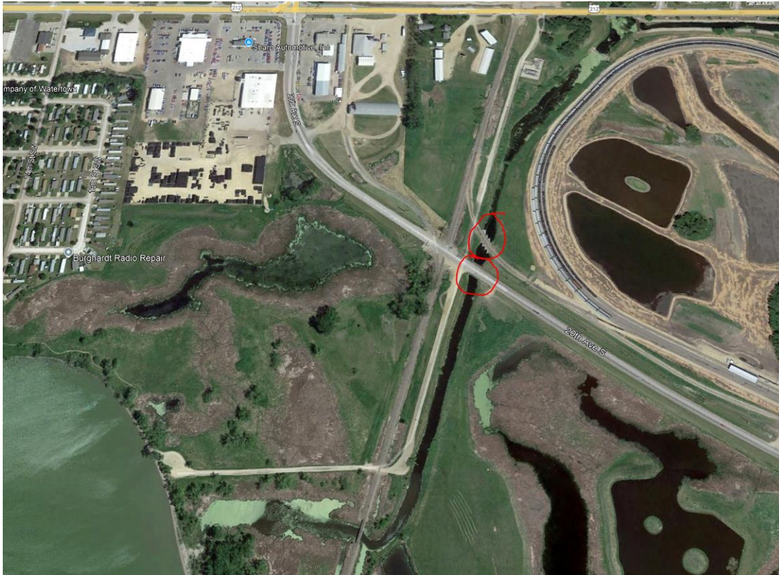
Tributary to Pelican Lake Branch Structures
