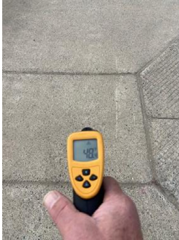
Figure 13 Sidewalk of adjacent street
