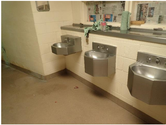
7. Lavatory with accessible dimensions
