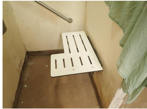
12. Non-compliant shower seat with wide section at front of compartment
