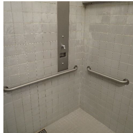
20. Compliant shower controls and grab bars
