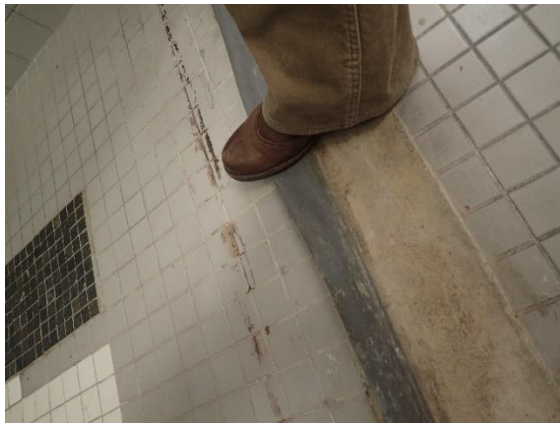
21. Flexible water dam at shower threshold
