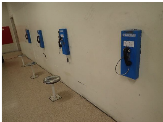
1. Telephone with compliant reach range
