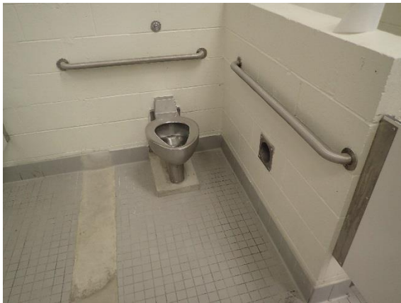
19. Accessible water closet and grab bars
