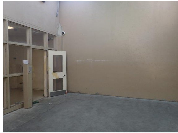
34. Call button is at above reach range, however was compliant when constructed.
