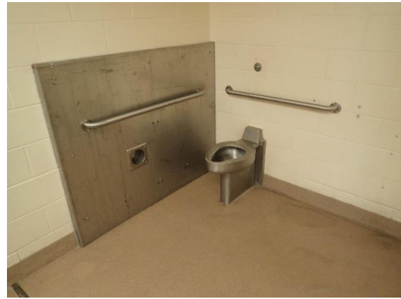
8. Water closet with compliant 18" between centerline and wall
