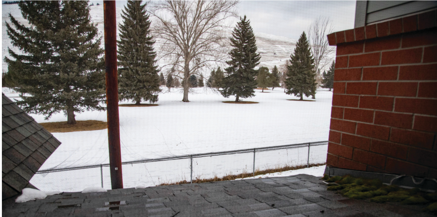
The view out of Meredith Iams' window. The screen was knocked out and is likely the path the intruders took to break in. EMMA SMITH | MONTANA KAIMIN
