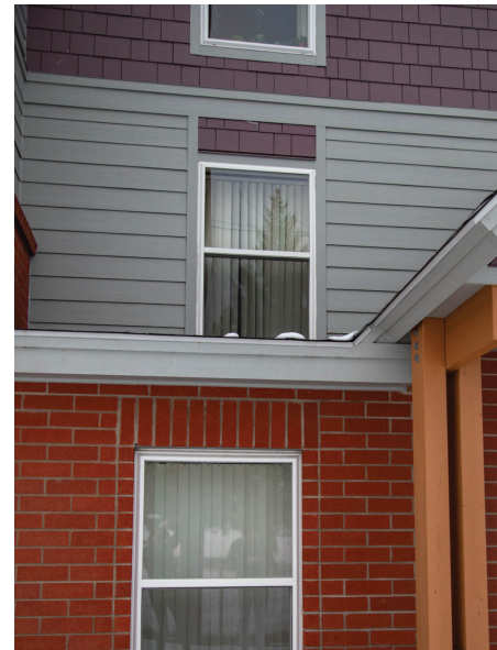
The window on the second floor of Lewis and Clark where the intruder possibly broke in. Residents believe the intruder climbed up the beam and pulled themselves onto the roof. The window was open. EMMA SMITH | MONTANA KAIMIN
