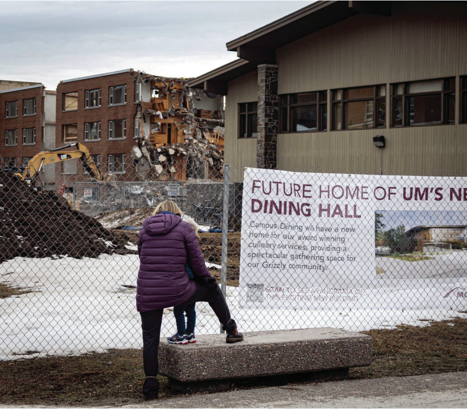
Desks and beds hang out of what once was the north end of Craig Hall while a mother and her son watch the demolition on Feb. 8. The area around Craig Hall is one of a few demolition sites planned for a newly renovated dining hall and remains blocked off, forcing students to take alternative routes to get around the construction site. Dining hall renovations are projected to start in early March. RIDLEY HUDSON | MONTANA KAIMIN
