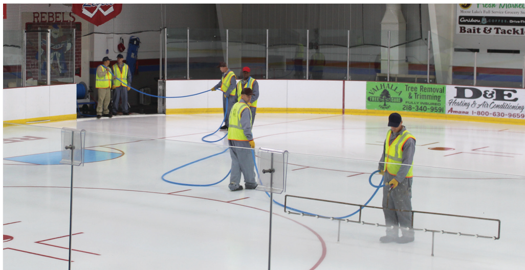
Ice at Riverside Arena in Moose Lake is going in. Above, Guyal Nelson and his assistants from the Willow River Challenge Incarceration Program work to create thin layers of water that freeze to create smooth skating ice.
