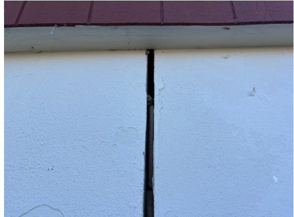
Figure 8 – Deteriorated sealant
