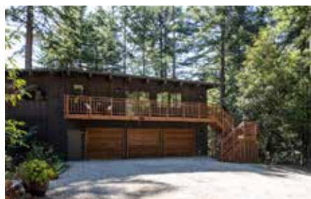
160 Redland Road, Woodside
