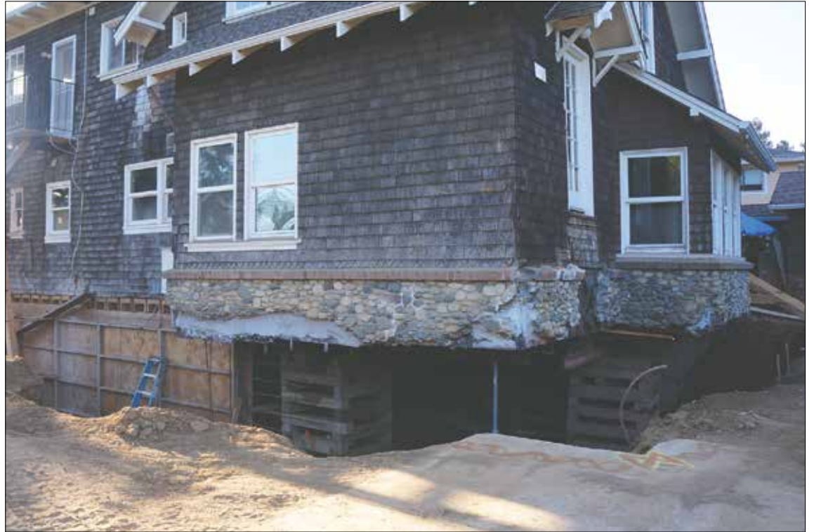
The Reouk family lofted their historical farmhouse to rebuild a foundation on the way to updating its interior.
