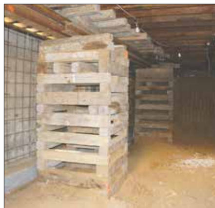
The Reouk family lofted their historical farmhouse to rebuild a foundation on the way to updating its interior.
