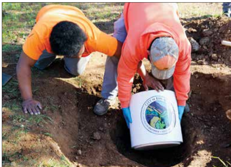
City workers prepare to place a time capsule in a prepared hole at the new Los Altos Community Center site.
