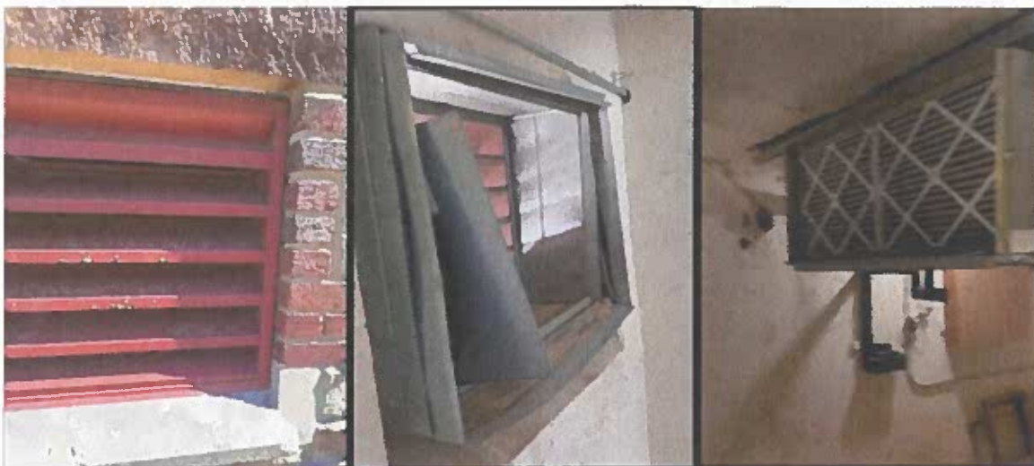
The “repaired” Johnson Hall air intake system on October 10, 2024. The ductwork (middle) between the outside, red vent (left) and the air intake (right) is detached and the air intake filter was moldy and unclear.
