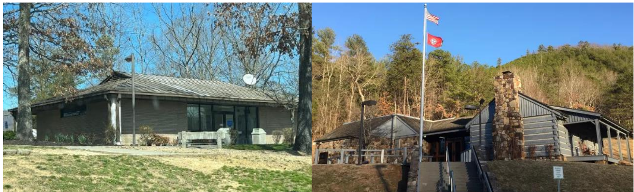
Figure 20 I-81 Greene County Rest Area Southbound (Left) and I-40 Smith County Welcome Center
