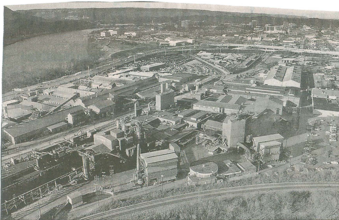
Wheland Foundry stretches out near the Tennessee River.
