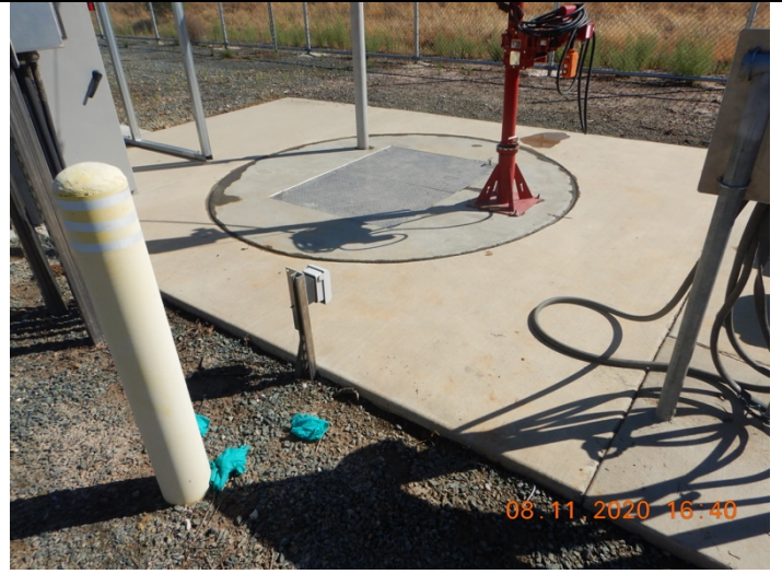
Photo 2. Vault of lift station where overflow occurred. Knife gate in photo 1 is approximately 20 feet to the right. Vault is approximately 500 feet from the creek bed of Mule Creek.
