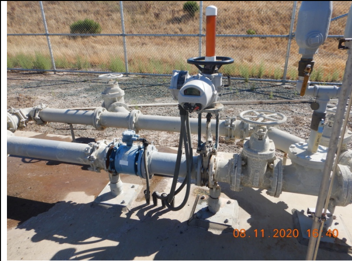
Photo 1. Knife gate that was closed by SCADA system failure, causing the backup in the lift station vault and eventual overflow. Lift station is located just southwest of Mule Creek Infill Complex.
