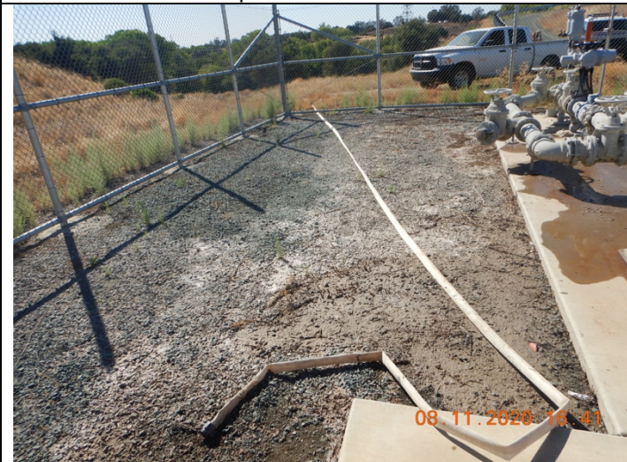
Photo 3. Hose running from small diversion downhill from the lift station back to the lift station vault. Hose was used to pump back collected sewage in bermed area (see photo 4).
