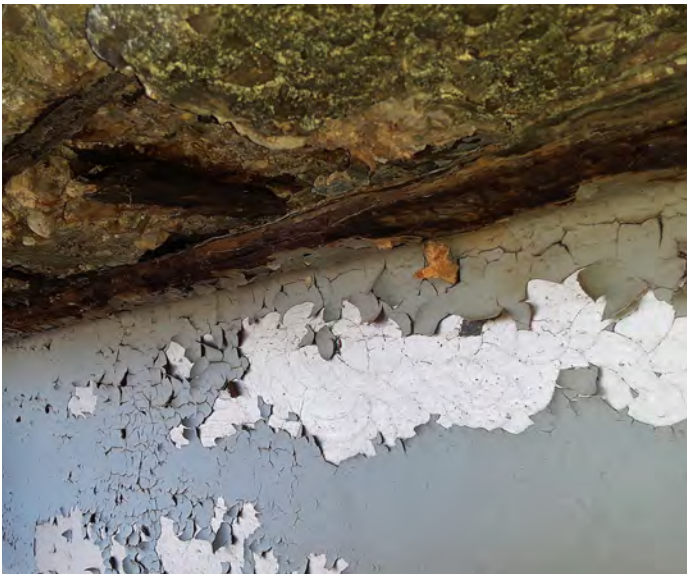
Close-up of severe corrosion.
