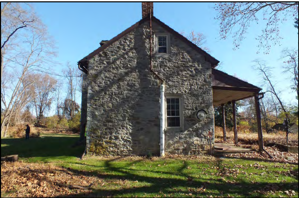
Photograph 6. West elevation (side) of the west addition, facing east (November 2023).
