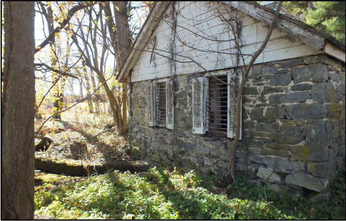
Photograph 17. East elevation (back) of the springhouse, facing southwest (November 2023).
