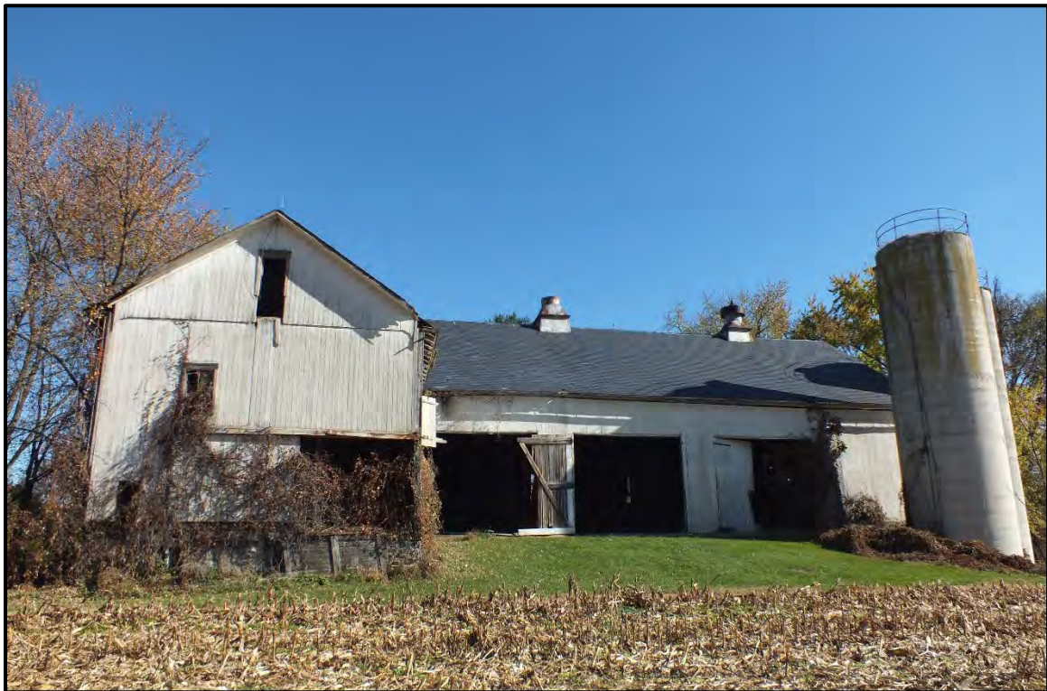
Photograph 26. West façade of the Pennsylvania Barn, facing northeast (November 2023).
