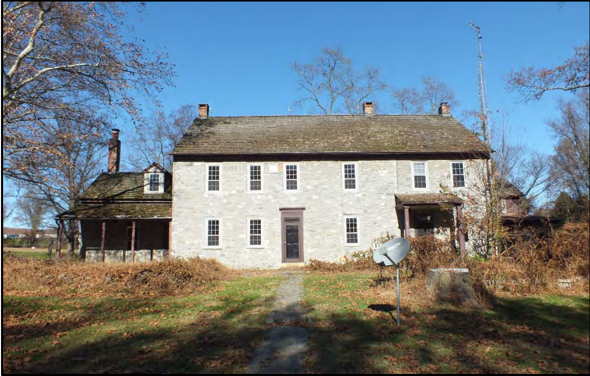
Photograph 1. South façade of the farmhouse, facing north (November 2023).
