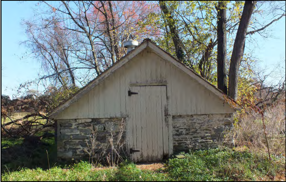
Photograph 15. West façade of the springhouse, facing northeast (November 2023).
