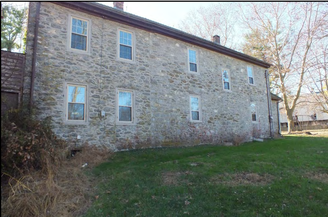
Photograph 4. North elevation (back) of the farmhouse, facing southwest (November 2023).
