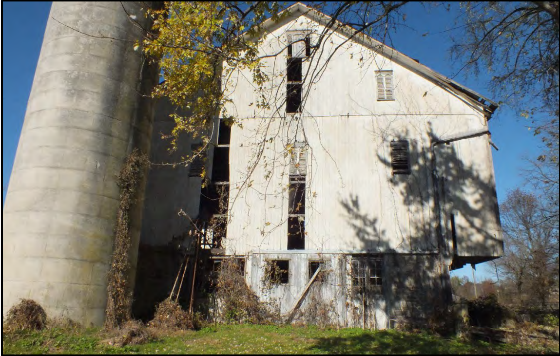
Photograph 29. South elevation (side) of the Pennsylvania Barn, facing northwest (November 2023).
