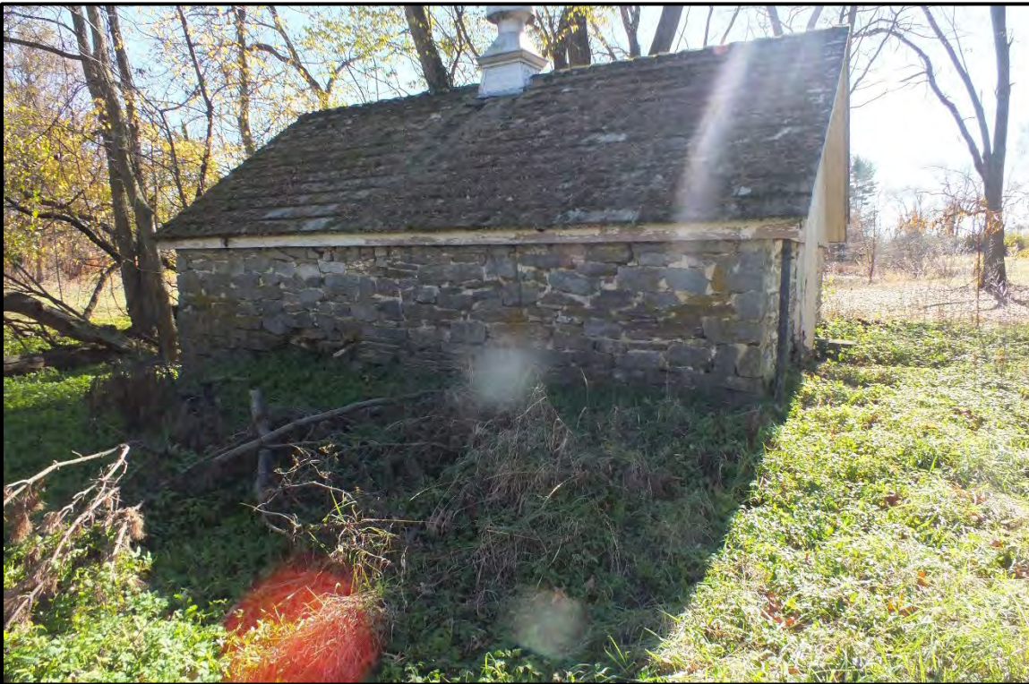
Photograph 16. North elevation (side) of the springhouse, facing east (November 2023).
