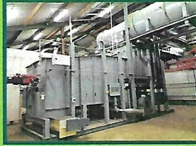
Swine Manure Netherlands Completed
