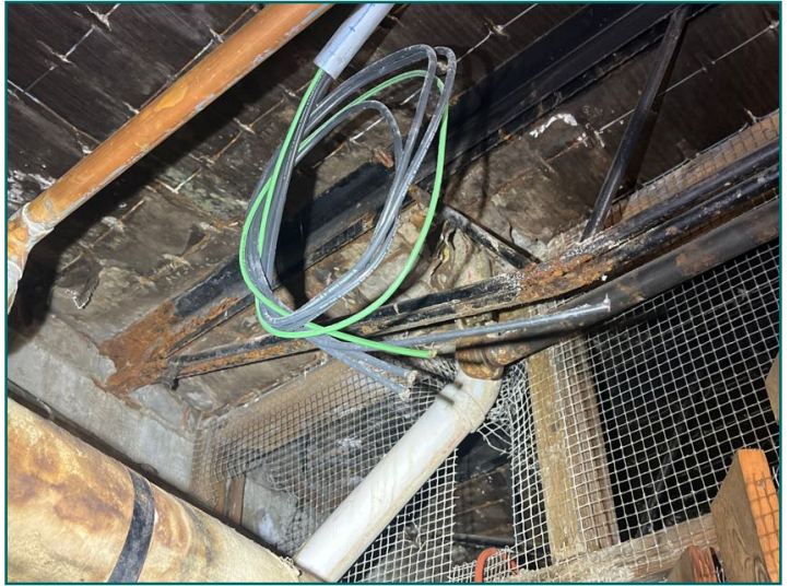
Corrosion on framing members at left side
