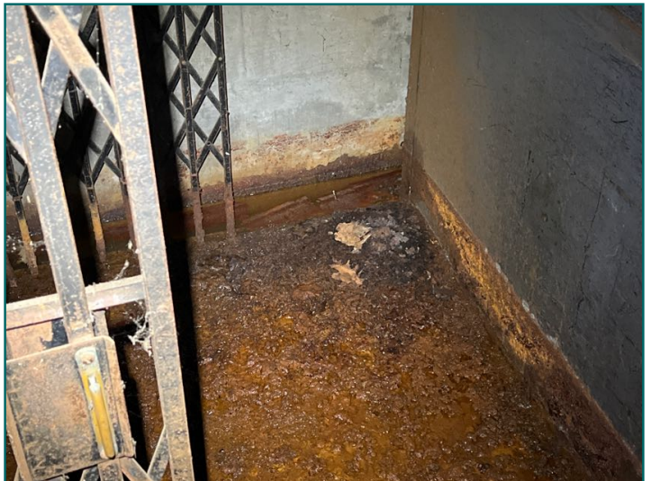
Elevator / elevator shaft are filled with water
