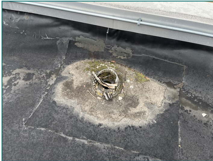
Damage roof drain cover
