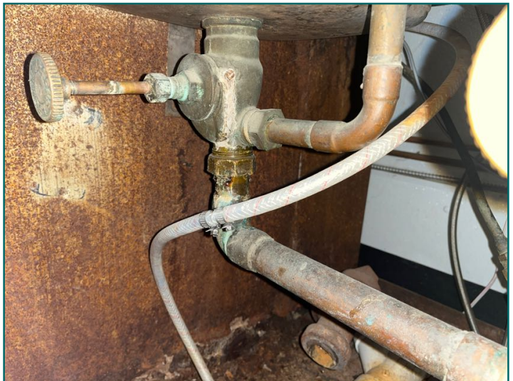
Corrosion / suspected leak on fittings below sink at left side / kitchen
