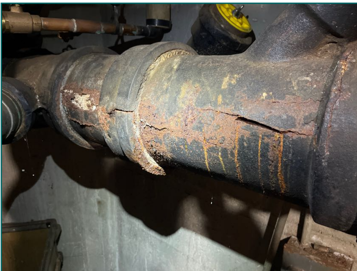
Cracked / damaged drain pipe at left side
