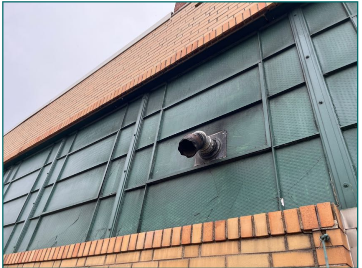
Pellet stove vent termination at right side
