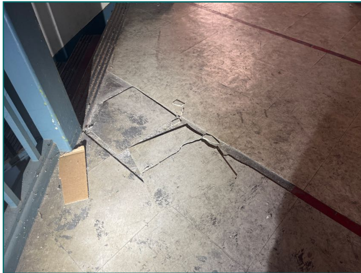
Cracked / damaged tiles at rear
