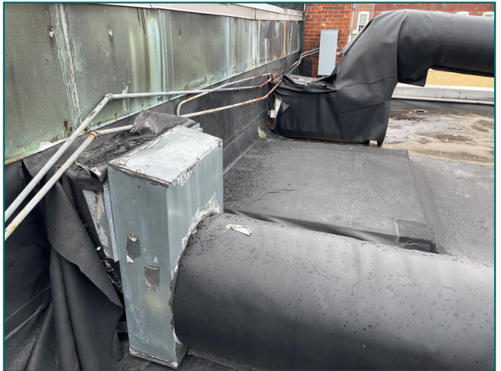
Damaged flashing around HVAC penetrations
