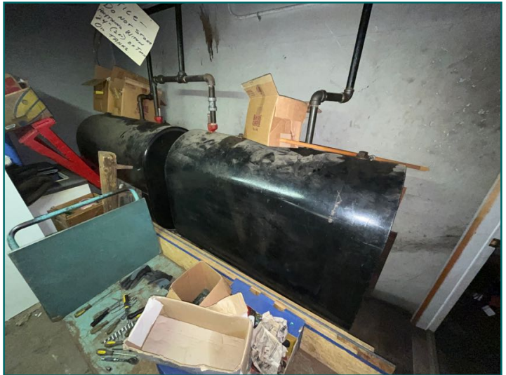
Dry oil stains / corrosion on tank noted
