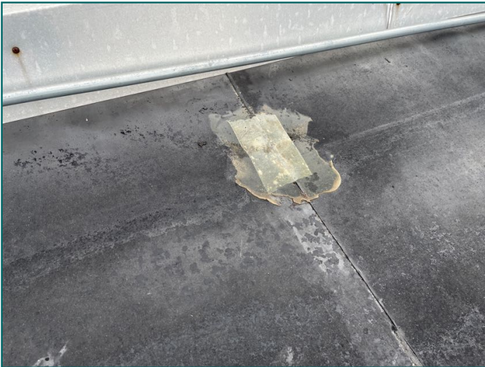
Numerous patches / repairs noted to roof surface
