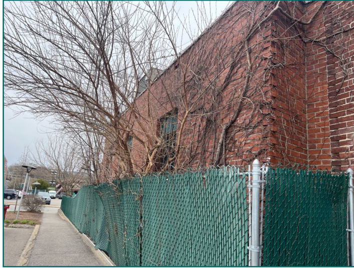
Vegetation in contact with siding at rear of building
