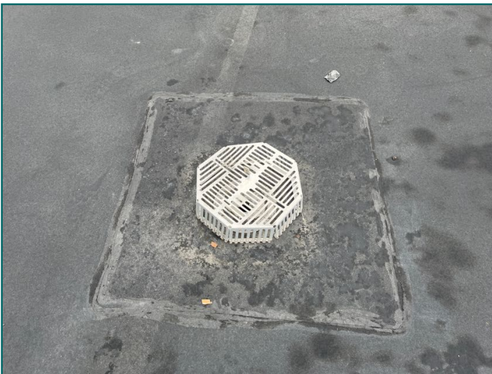
Internal roof drains throughout
