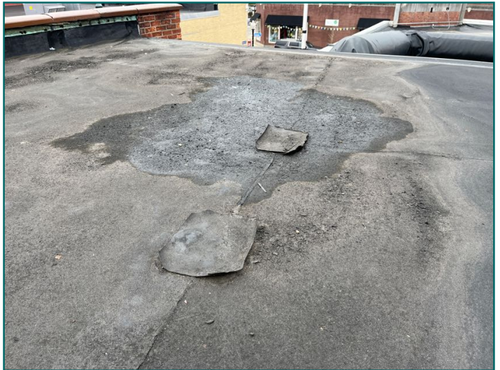
Damaged / lifting patches on rear roof surface
