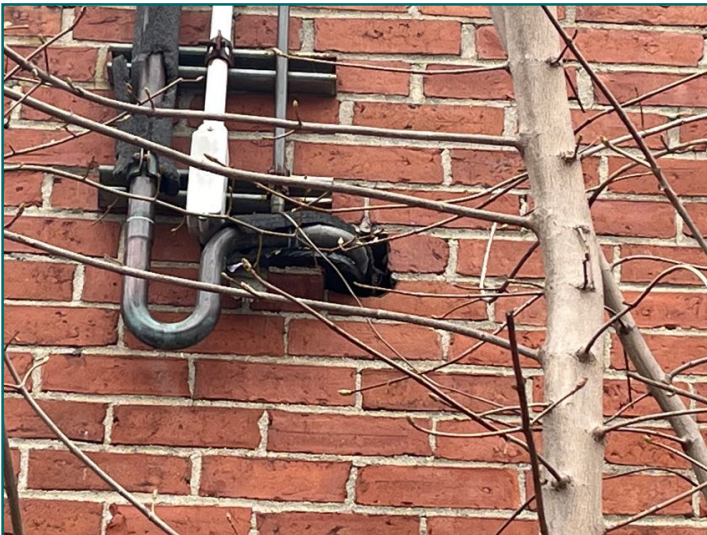
Penetration gaps at rear
