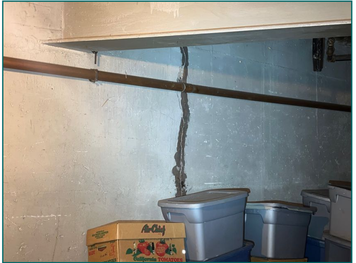
Vertical crack on front wall with repairs
