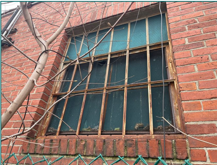
Corrosion on frame at rear
