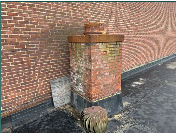
Deterioration to brick and grout
