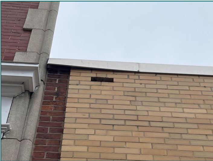
Damaged / missing brick at front
