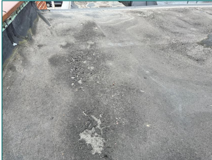
Deterioration to rear roof surface
