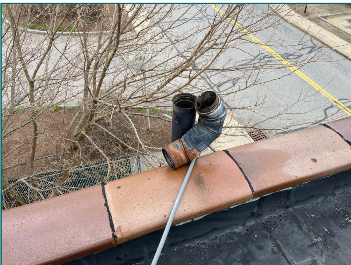
Vent termination at rear is damaged
