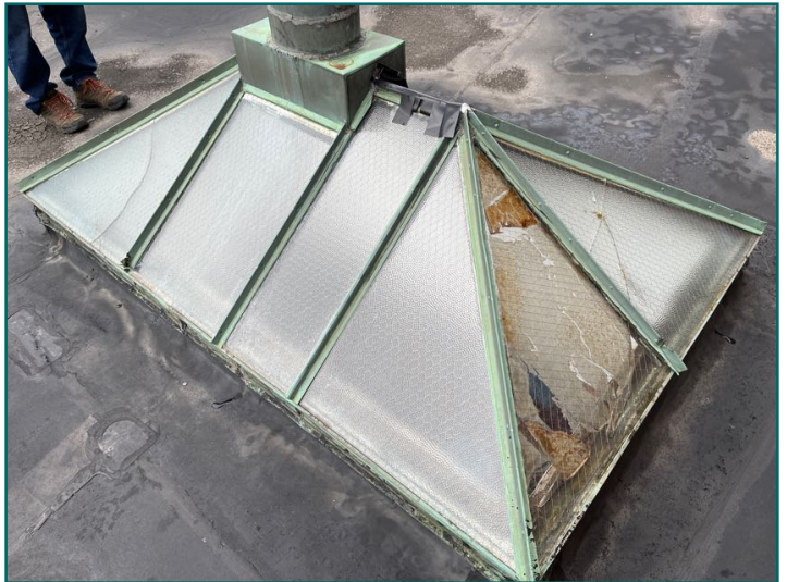
Damaged skylight / broken glass at rear
