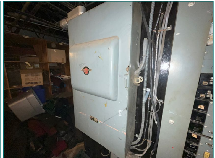
Main electrical disconnect
