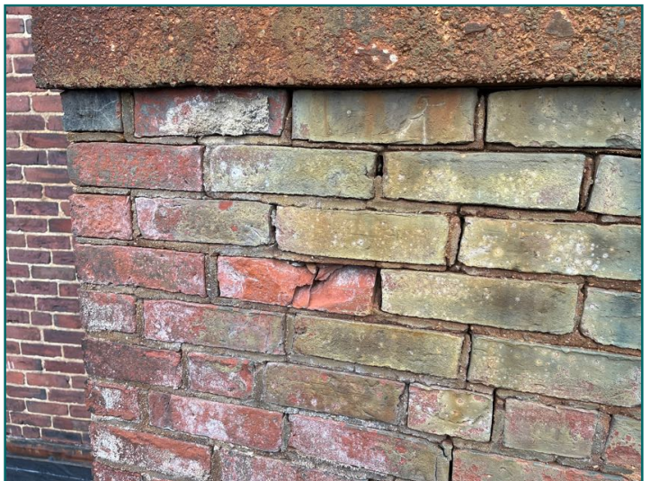
Deterioration to brick and grout
