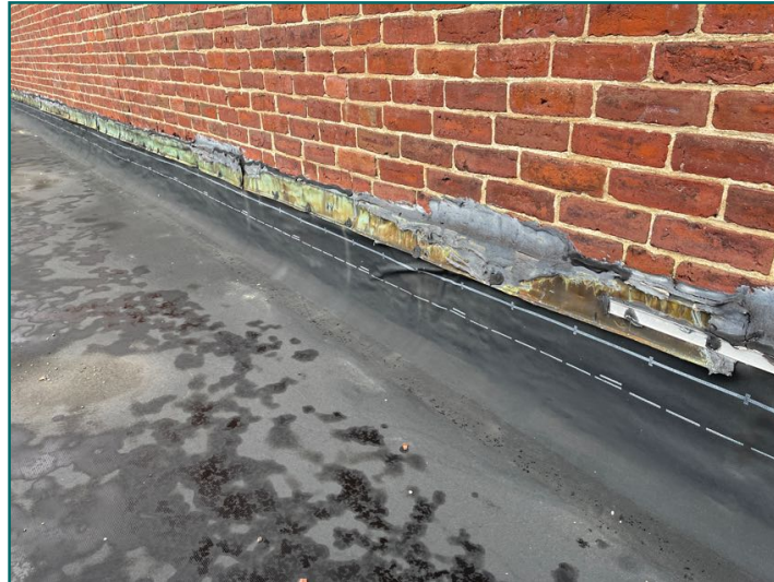
Dried / cracking flashing sealant at shared wall
