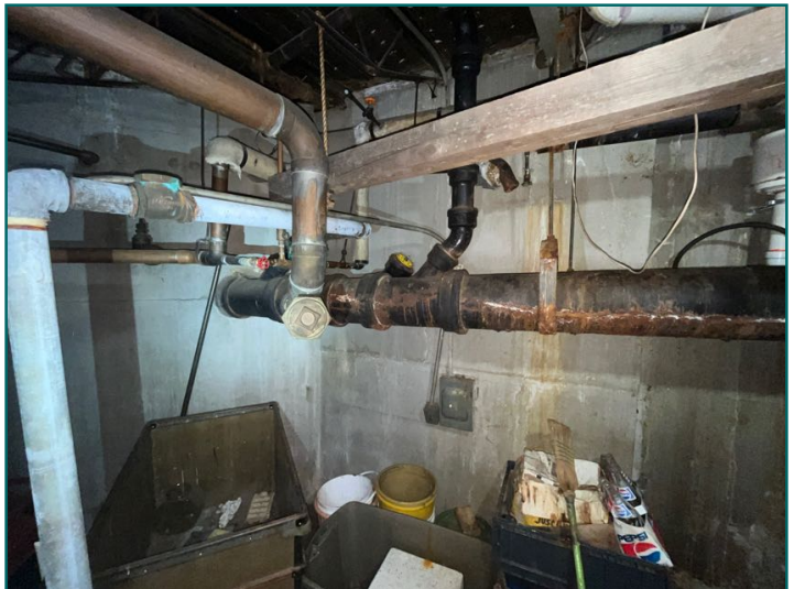
Main drain line termination
