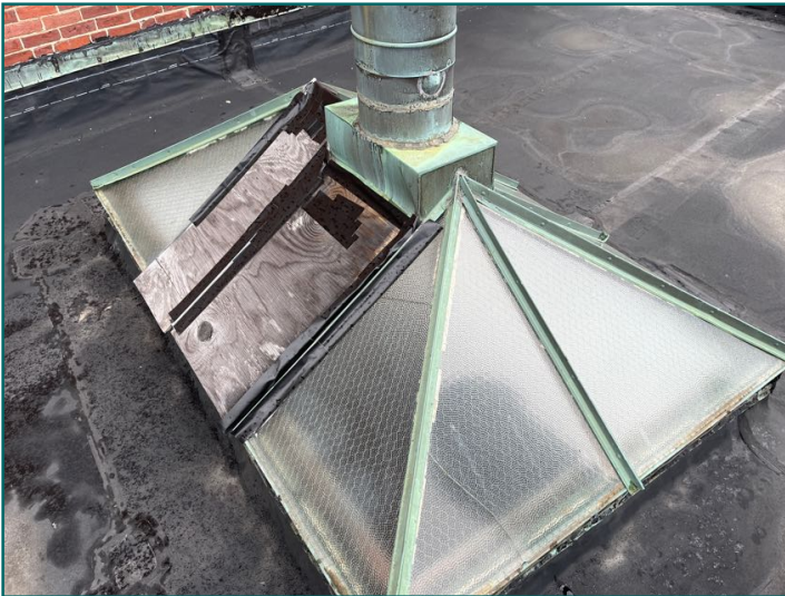
Damaged skylight / broken glass at rear
