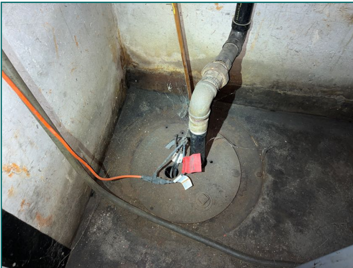
Sump pump at rear of basement, drain termination not located.
