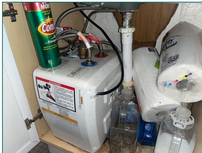
Electric water heater in first floor bathroom, age not determined
