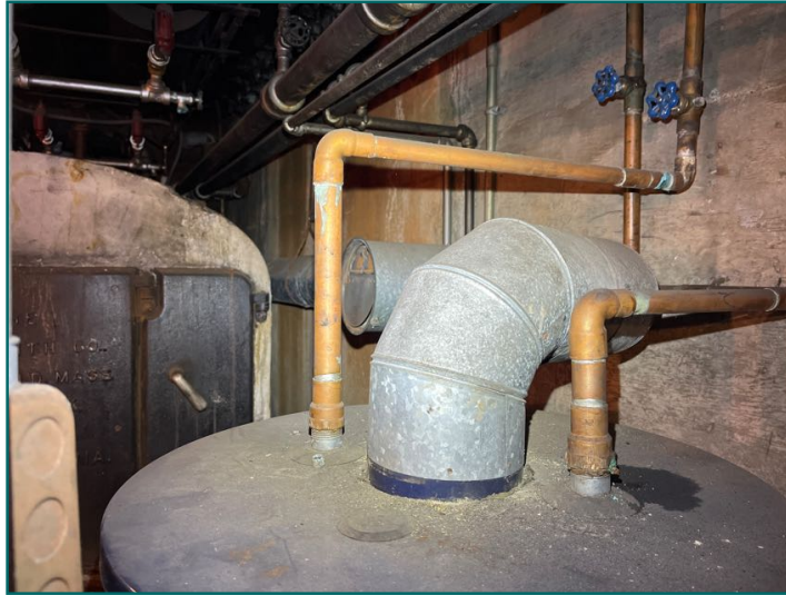
Water heater is gravity vented
