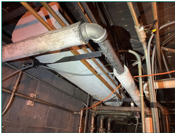
Suspected Asbestos insulation on boiler distribution noted
