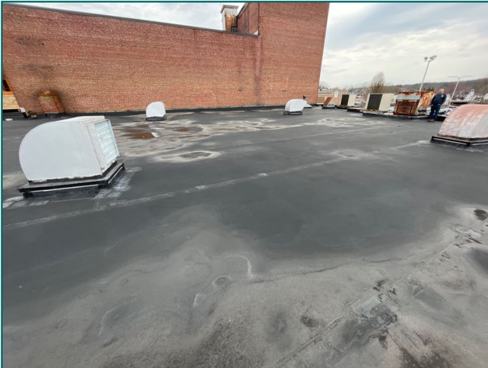
HVAC vent terminations on roof
