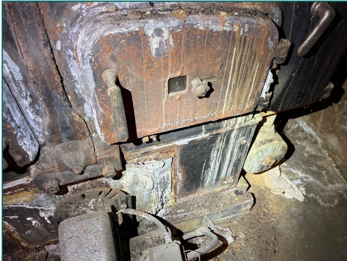
Corrosion on boiler noted
