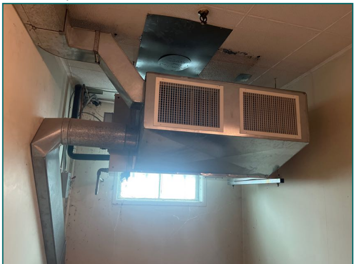
Air handler at rear stairwell, age not determined
