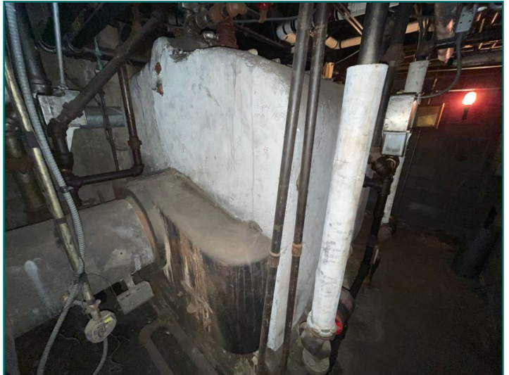
Suspected asbestos insulation on boiler
