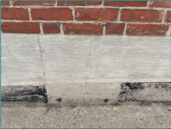
Vertical crack on side wall.
