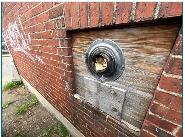
Vent termination at rear is sealed / no longer in use
