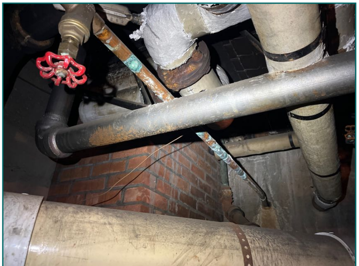
Corrosion on fittings at left side
