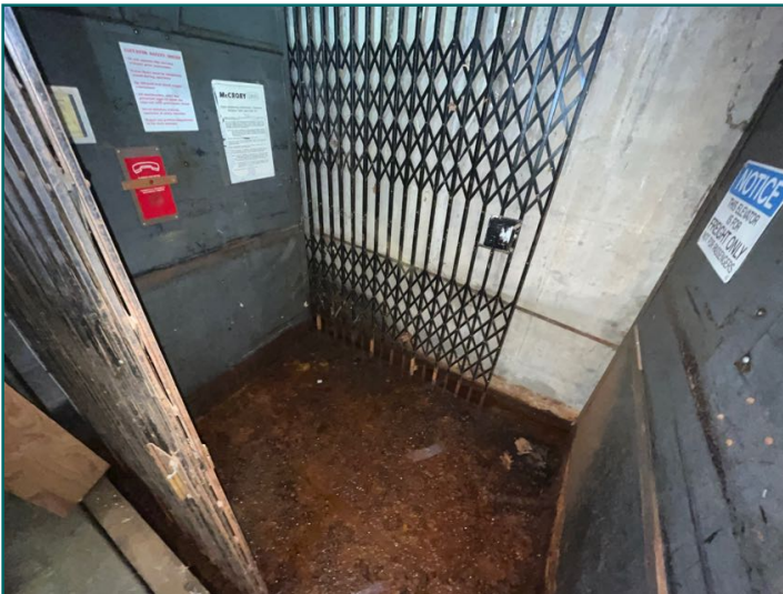
Elevator / elevator shaft are filled with water
