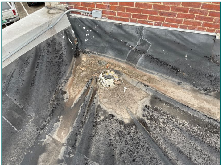
Damage roof drain cover
