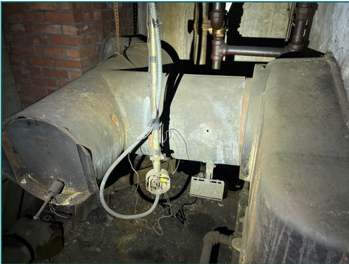
Boiler vent termination
