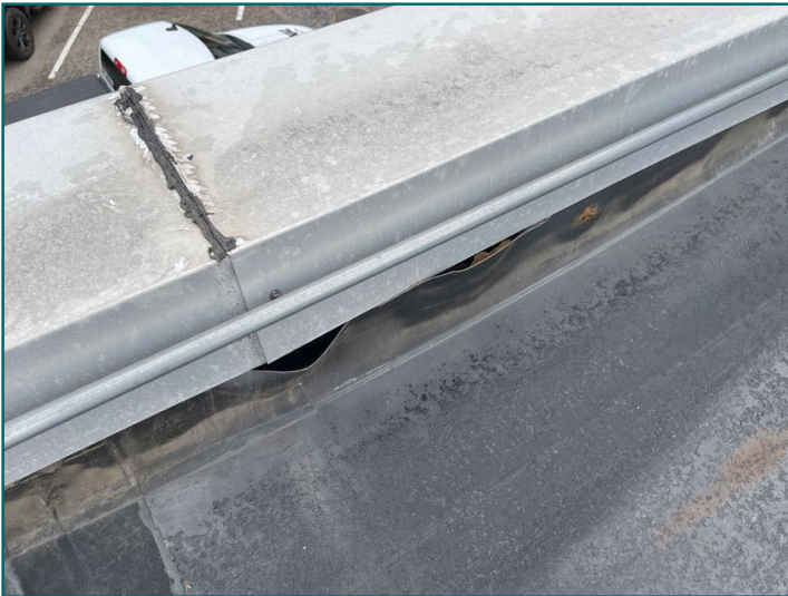
Sections of damaged flashing at front
