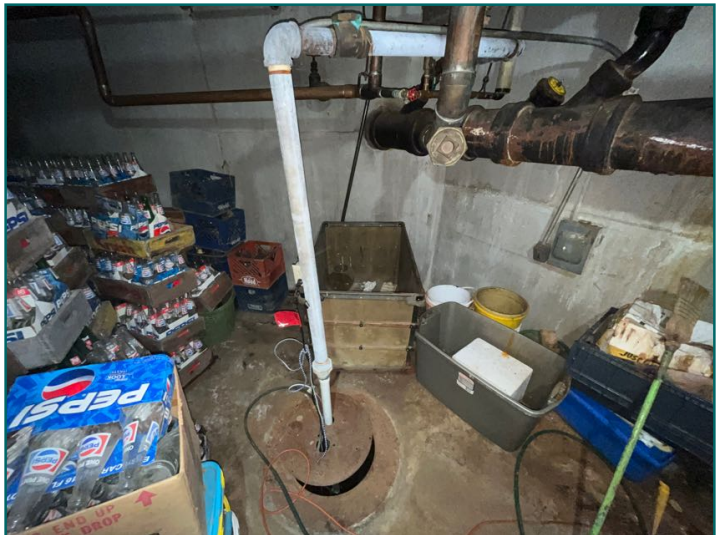
Sump pump at front of basement drains into sewer system
