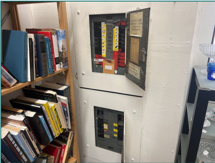
Sub panels at right side first floor
