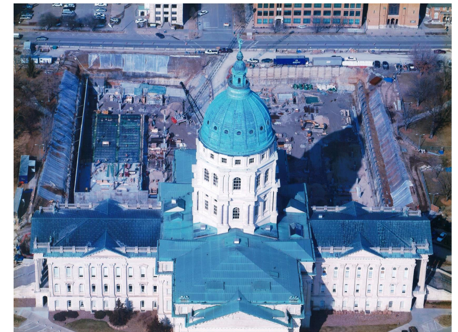
Example of lagging system of excavation. Kansas State Capitol.
