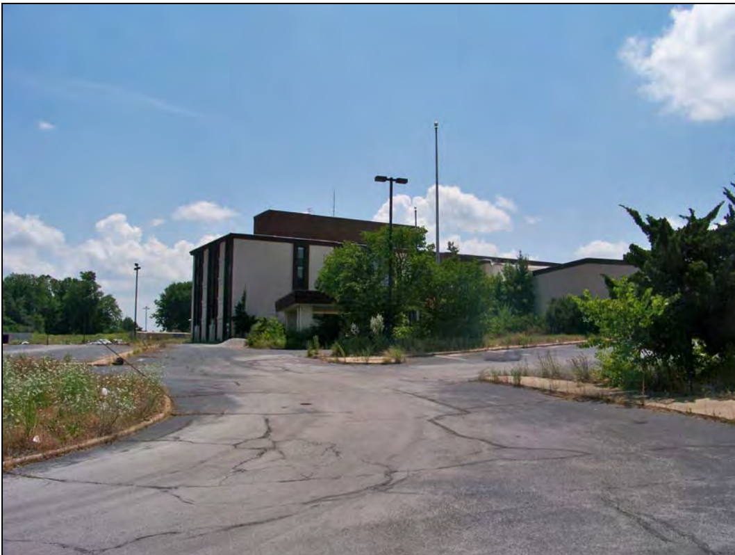
Parcel No. 04-4.0-19-000-000-005.003 – looking east – overgrown vegetation; debris
