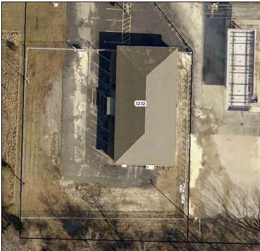
3232 E. 32 nd St – aerial – poor internal circulation (dead-end parking aisle)
