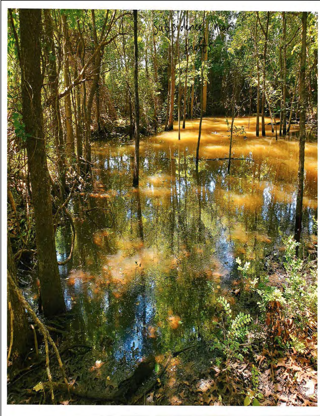
Parcel No. 04-4.0-19-000-000-005.000 – flooded area of subsidence near mine shaft
