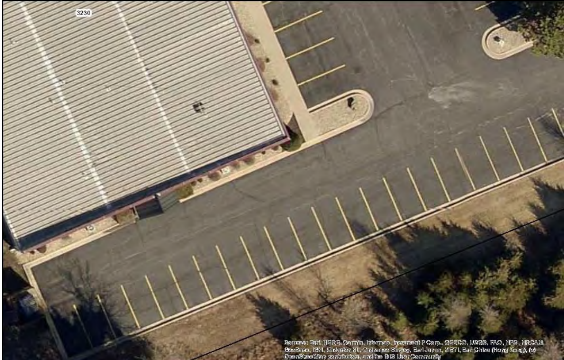
3232 S. Hammons Blvd – aerial – poor internal circulation (dead-end parking aisle)
