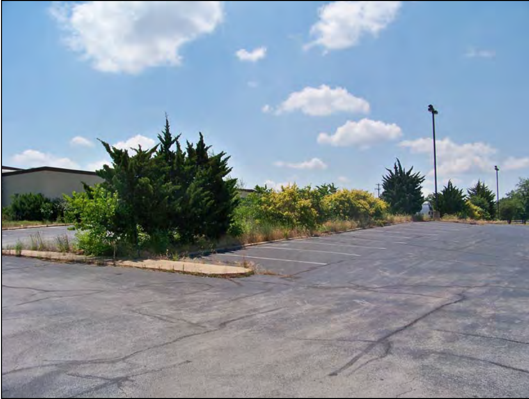
Parcel No. 04-4.0-19-000-000-005.003 – looking southeast – overgrown vegetation
