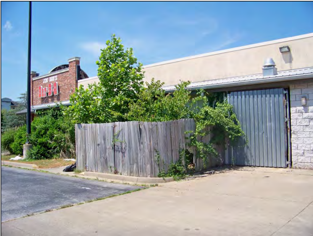
Parcel No. 04-4.0-19-000-000-005.007 – looking southwest – overgrown vegetation; trash/debris
