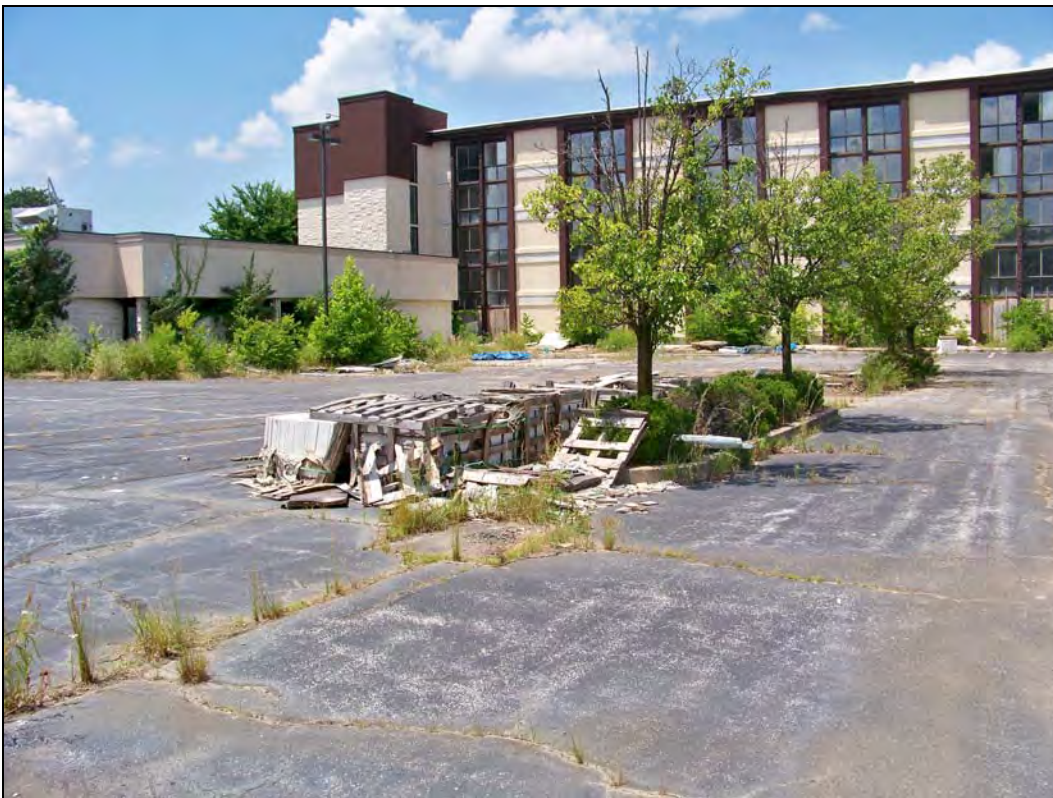
Parcel No. 04-4.0-19-000-000-005.003 – looking west – trash/debris; overgrown vegetation; deterioration of parking surface
