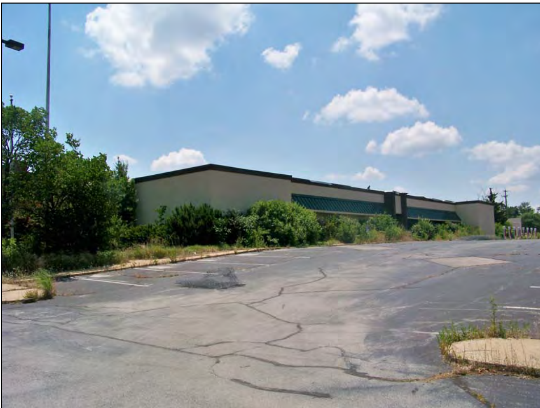
Parcel No. 04-4.0-19-000-000-005.003 – looking southeast – overgrown vegetation; debris
