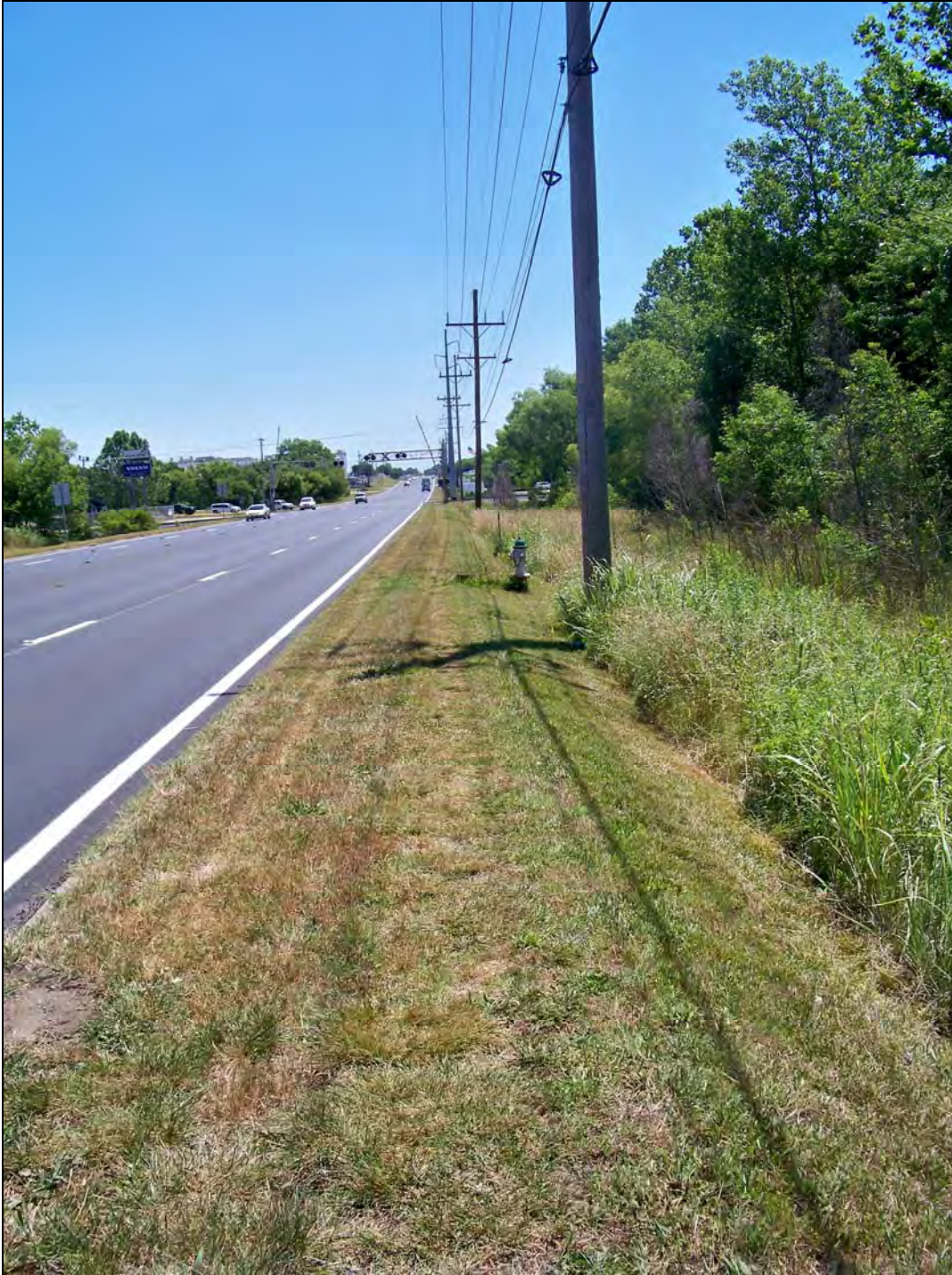
E. 32 nd Street – looking east – lack of pedestrian circulation; lack of curb/gutter
