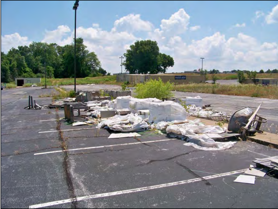
Parcel No. 04-4.0-19-000-000-005.003 – looking east – trash/debris; overgrown vegetation
