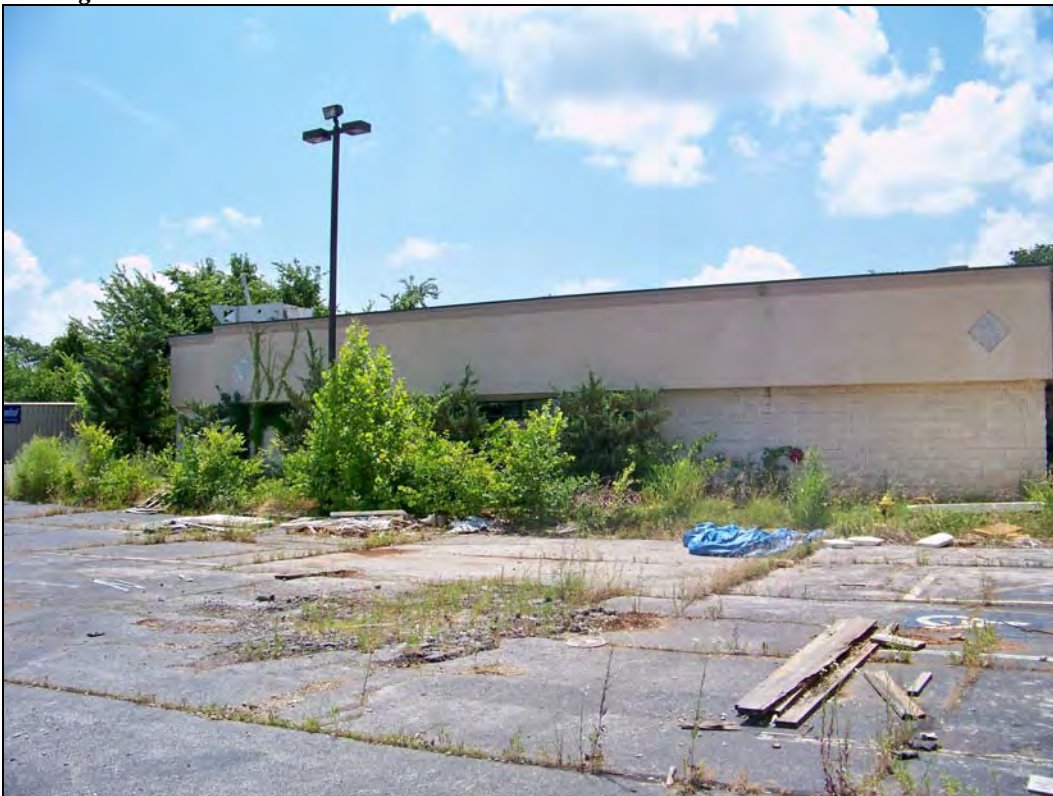
Parcel No. 04-4.0-19-000-000-005.003 – looking south – trash/debris; overgrown vegetation
