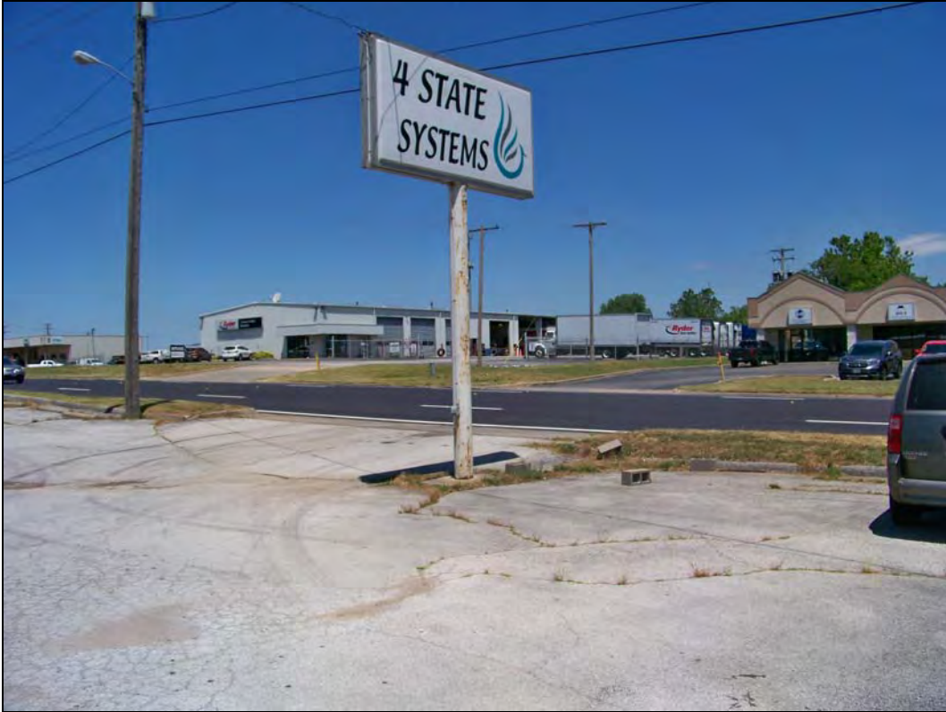
Parcel No. 04-4.0-19-000-000-006.000 – looking north – deterioration of pavement, sign
