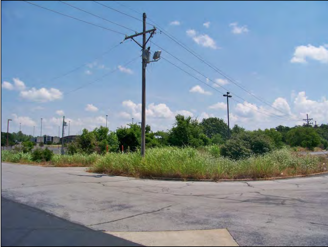
Parcel No. 04-4.0-19-000-000-005.003 – looking northeast – overgrown vegetation
