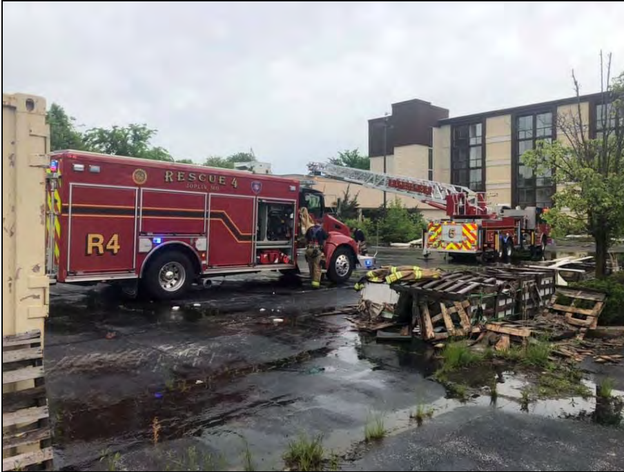
Joplin Hotel – Fire Department call to fire, May 15, 2020 (photo courtesy Joplin Fire Department)
