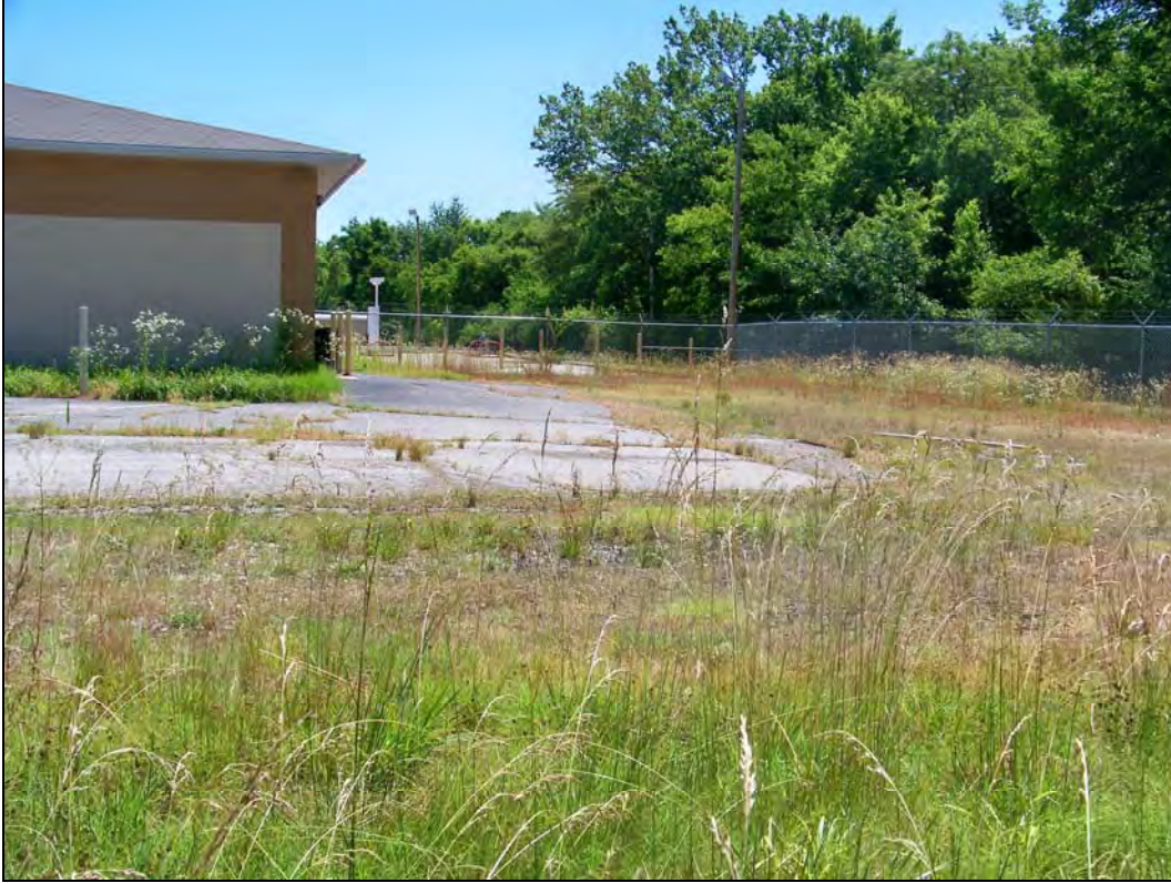
3232 E. 32 nd Street – looking east – overgrown vegetation; deterioration of parking lot
