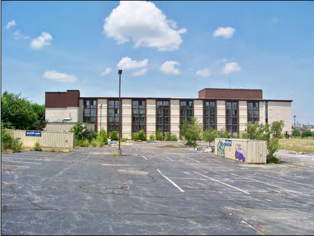
Parcel No. 04-4.0-19-000-000-005.003 – looking west – deterioration of pavement; graffiti
