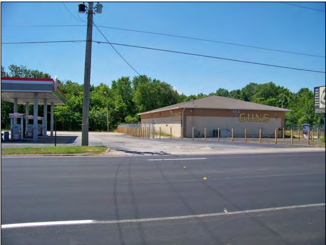
Parcel No. 04-4.0-19-000-000-005.007 – looking southwest – excessively wide driveway; no directional signage
