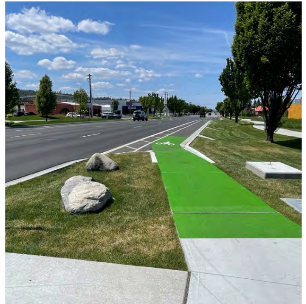
Sprague Avenue Buffered Bike Lane
