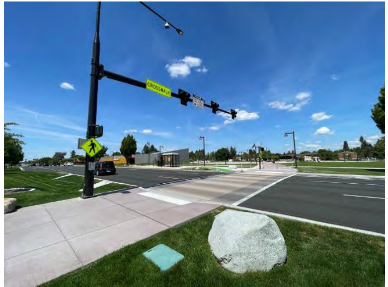
Sprague Avenue Crosswalk with Pedestrian Hybrid Beacon
